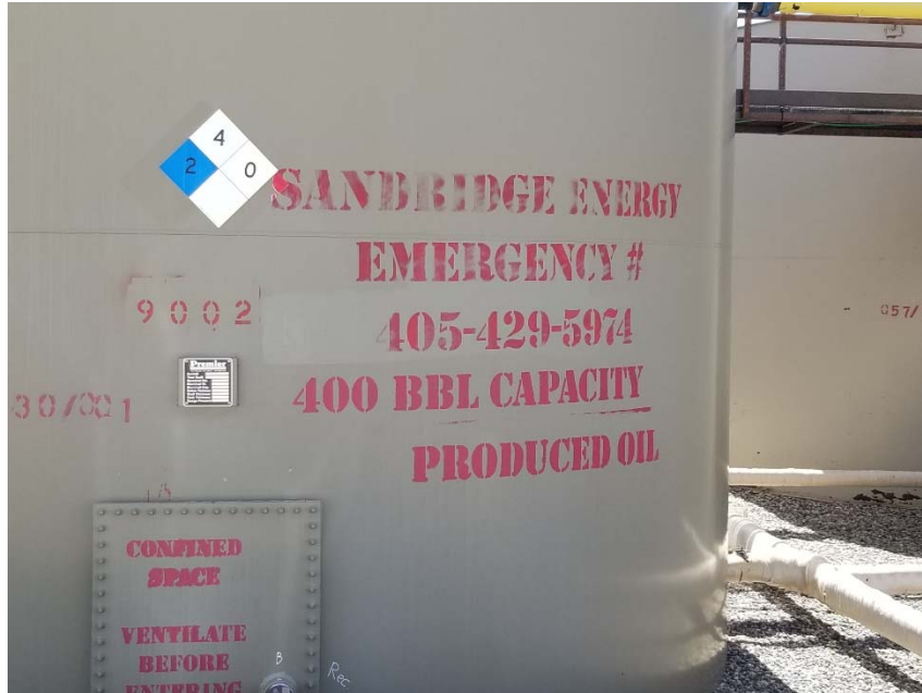
Photo 5. Tank label incomplete/inaccurate.
