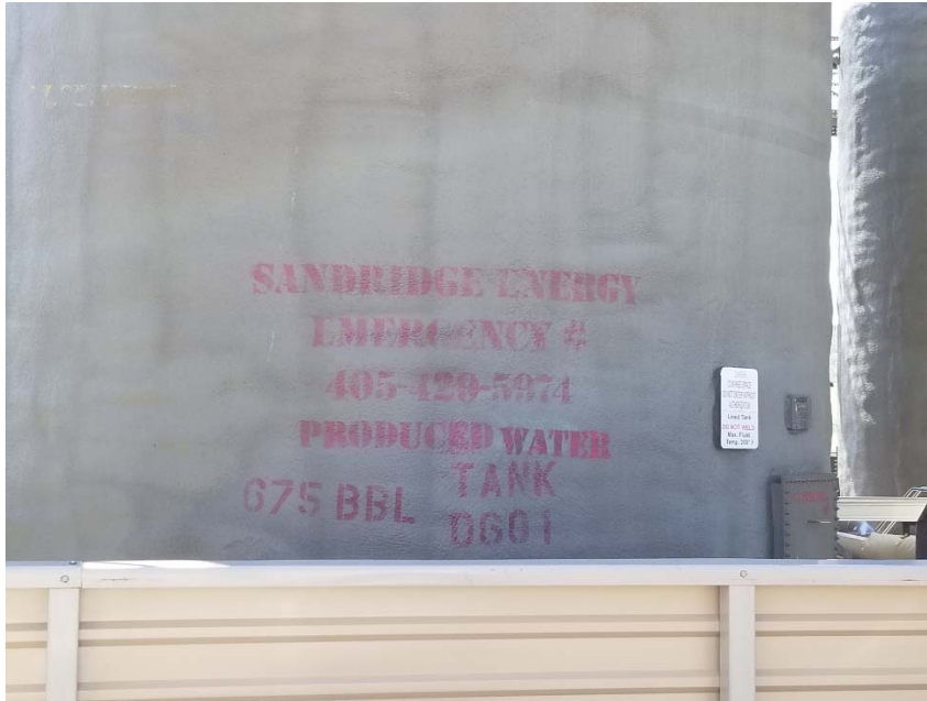
Photo 2. Inaccurate/incomplete tank labels.
