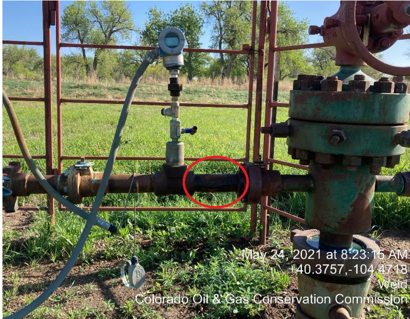
Photo #2 Split tubing on the casing side “mechanical conditions”
