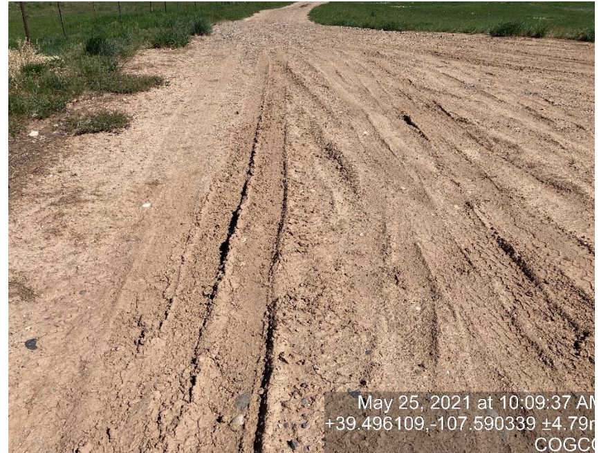
Lack of stabilization/compaction
