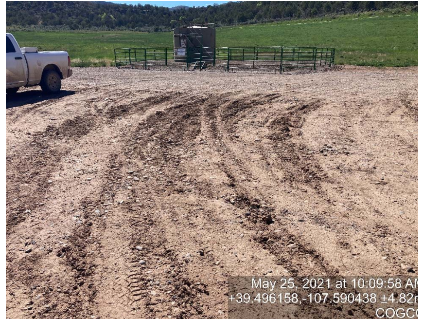
Lack of stabilization/compaction
