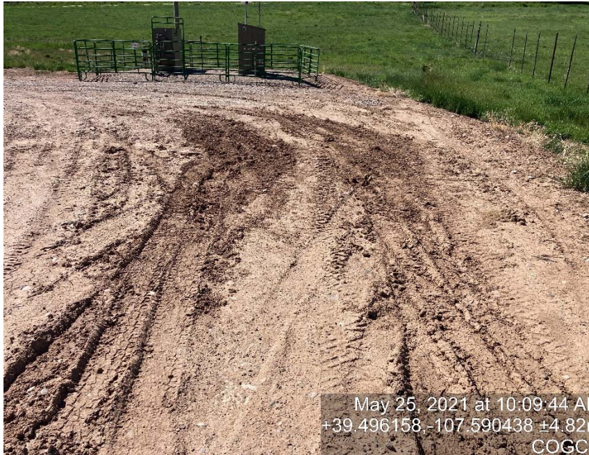
Lack of stabilization/compaction
