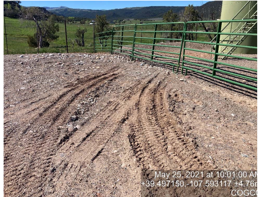
Lack of stabilization/compaction
