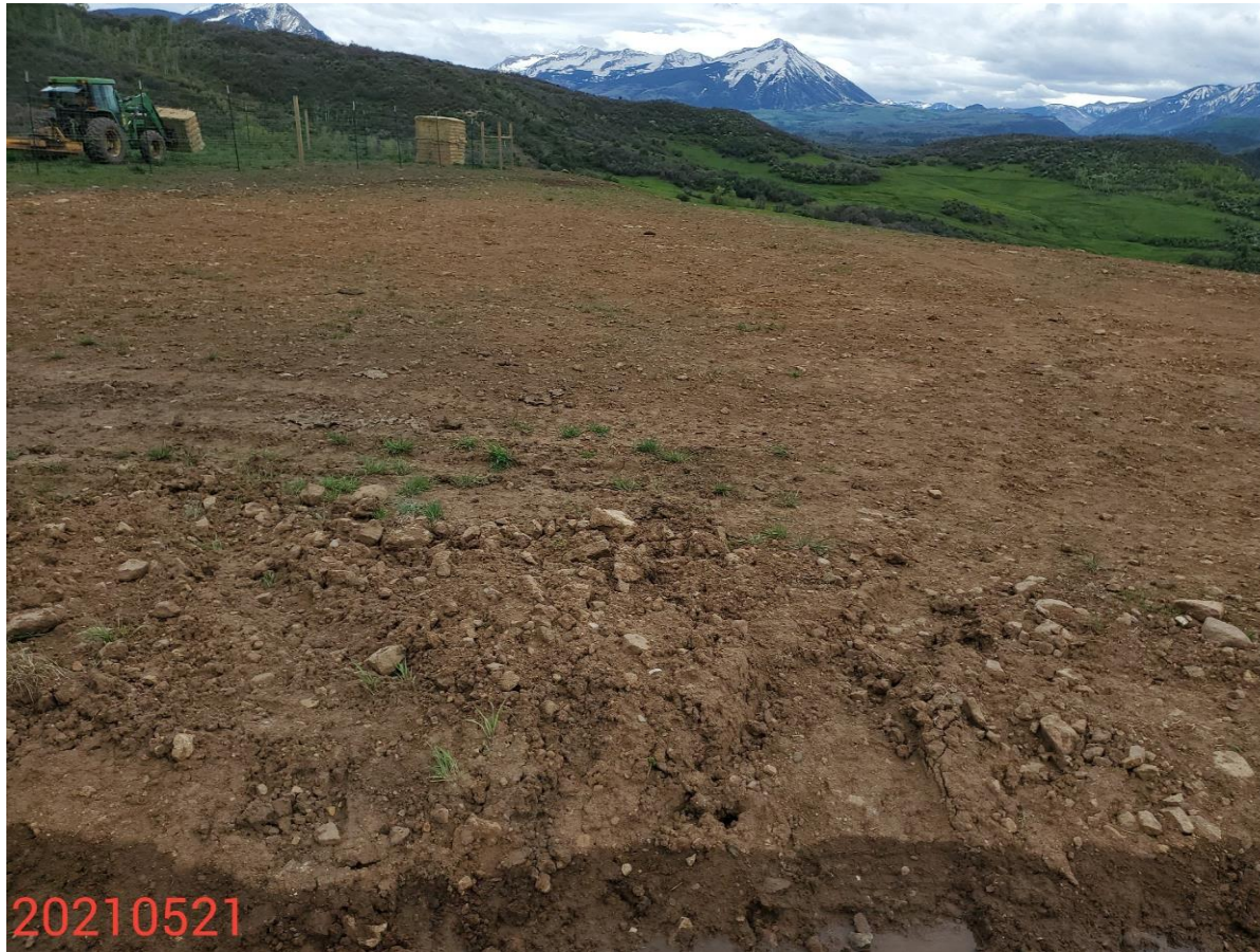
Photo 21: Photo taken northwest end of the Location, facing southeast. Photo shows control measures to protect/stabilize slopes and disturbed areas of the Location remain missing or insufficient; unable to find evidence that revegetation activities were performed, and BMPs to stabilize seeded soils implemented.
