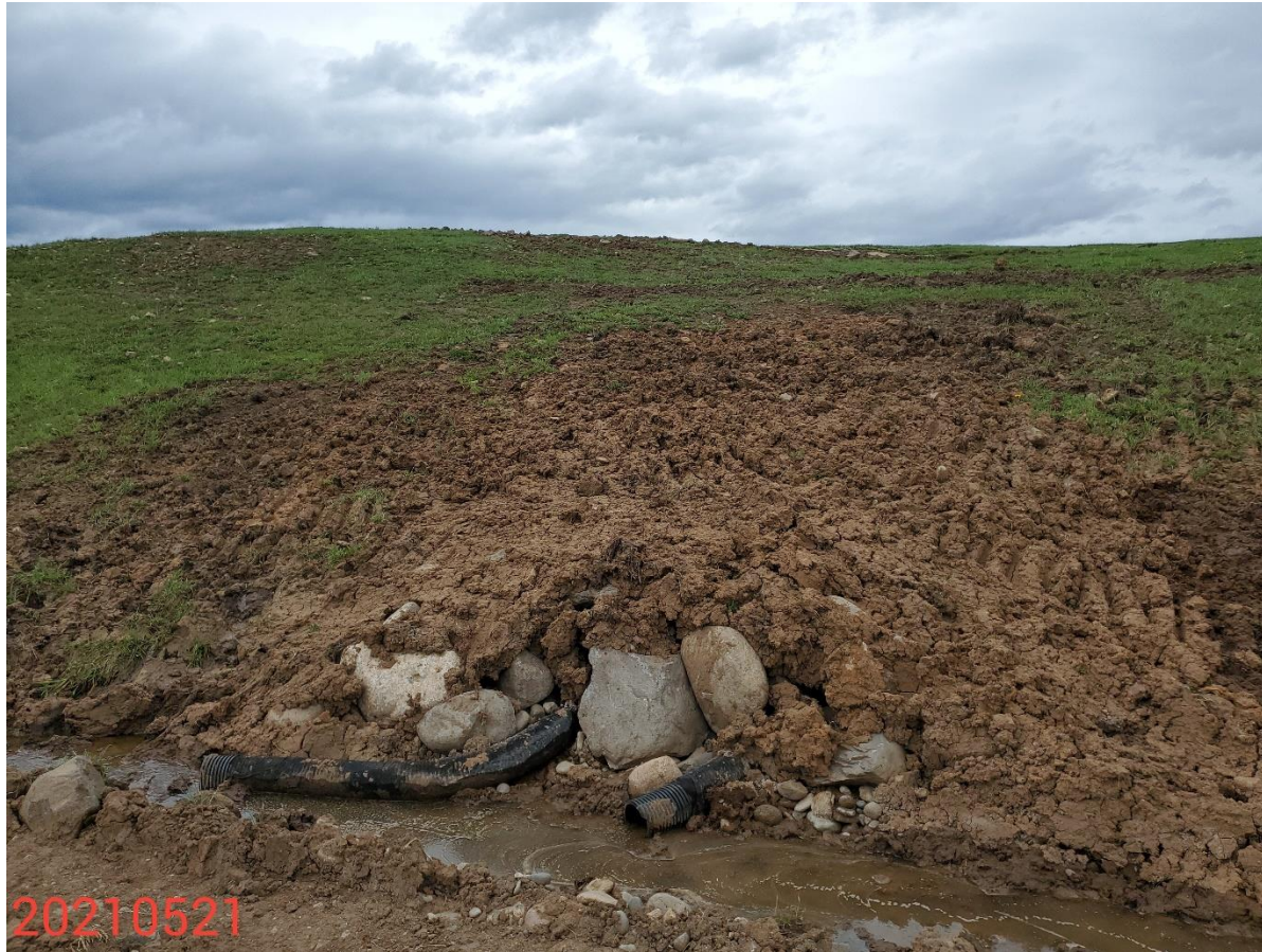
Photo 9: Photo taken from the north end of the Location, facing north. Photo shows control measures to protect/stabilize slopes and disturbed areas of the Location remain missing or insufficient. Unable to find evidence that revegetation activities were performed, and BMPs to stabilize seeded soils implemented.
