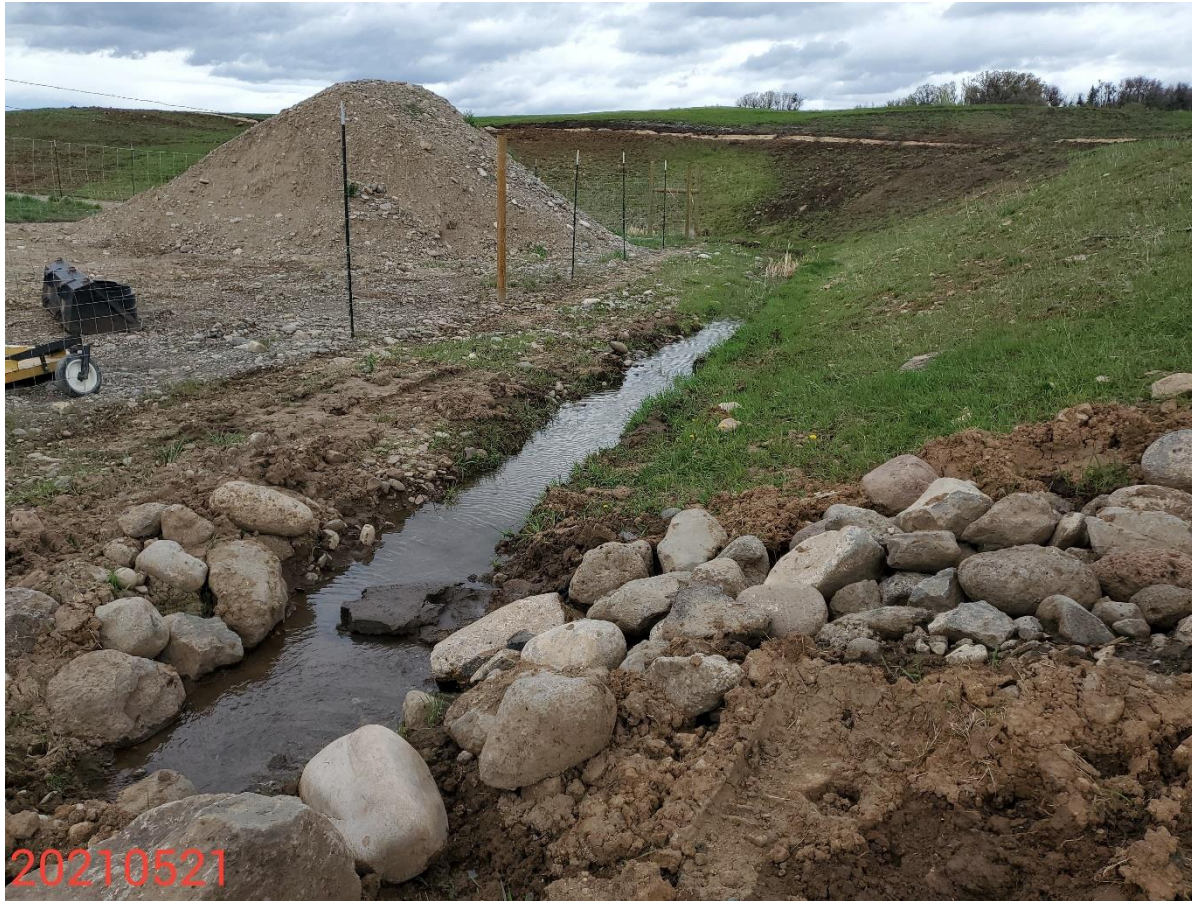
Photo 2: Photo taken from the east end of the Location, facing north. Photo shows the 2 nd stormwater diversion ditch around perimeter of the pad.
