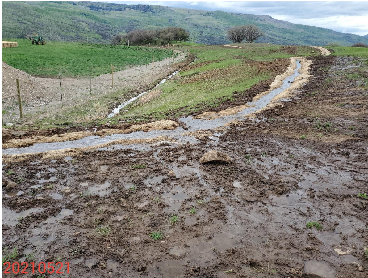
Photo 4: Photo taken from the northeast corner of the Location, facing southwest. Photo shows perimeter stormwater diversion ditch installed on Location is inadequate/insufficient for the site's conditions; diversion ditch not in proper functioning condition.
