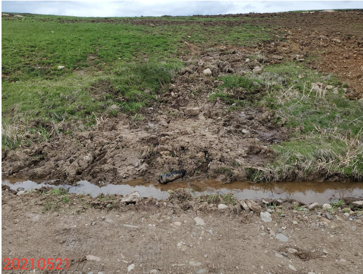
Photo 7: Photo taken from the north end of the Location, facing north. Photo shows control measures to protect/stabilize slopes and disturbed areas of the Location remain missing or insufficient. Unable to find evidence that revegetation activities were performed, and BMPs to stabilize seeded soils implemented.
