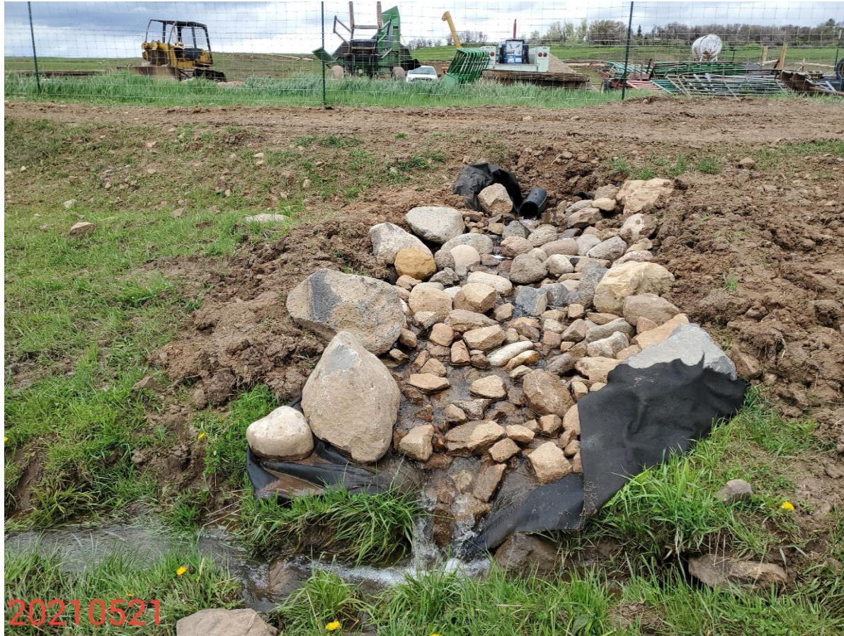
Photo 25: Photo taken from the ditch on the southeast end of the Location. Photo shows outlet protection of the stormwater diversion ditch has not been installed in accordance with good engineering practices; geotextile liner has been laid upon the soil rather than trenched in.
