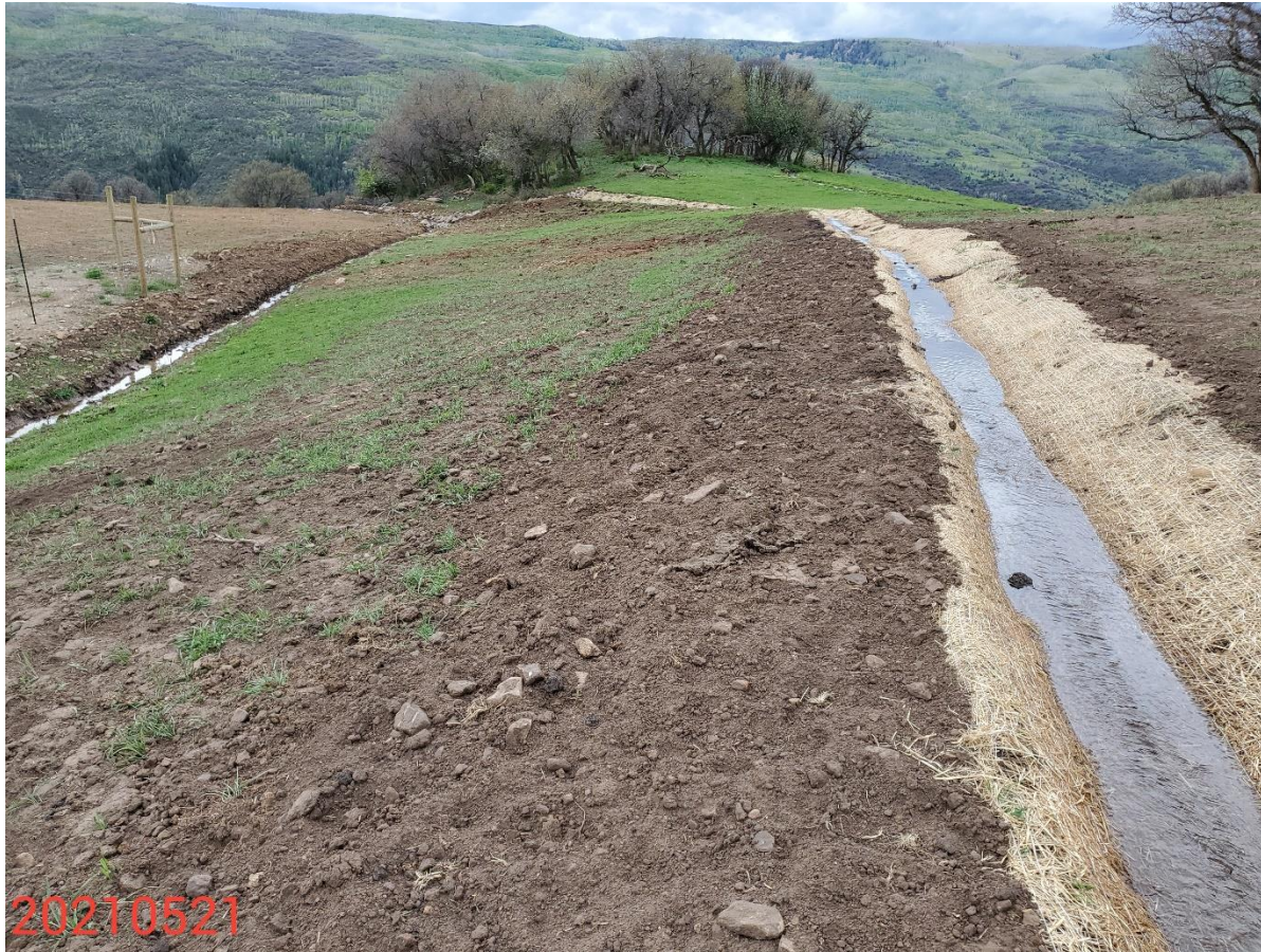
Photo 12: Photo taken from the north end of the Location, facing west. Photo shows stormwater diversion ditch constructed along perimeter of the Location.
