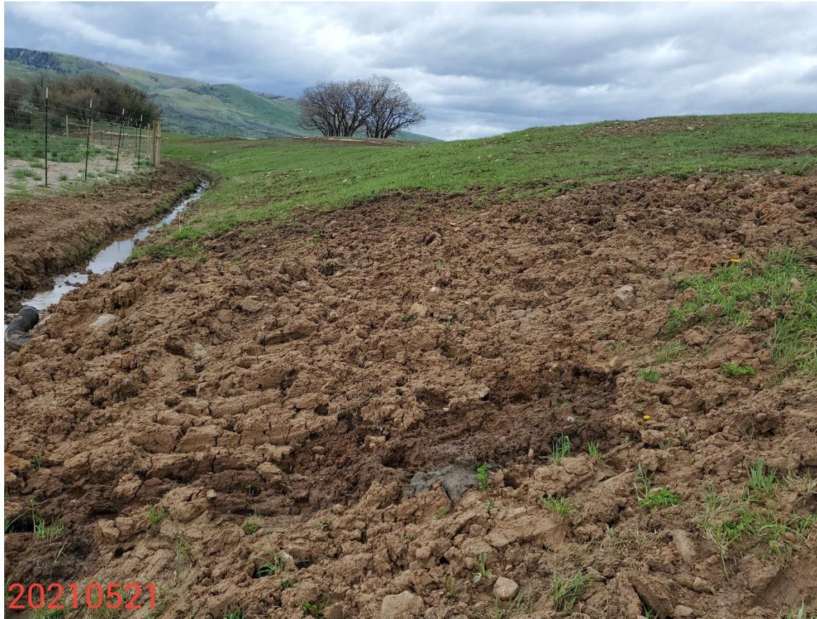
Photo 8: Photo taken from the north end of the Location, facing west. Photo shows control measures to protect/stabilize slopes and disturbed areas of the Location remain missing or insufficient. Unable to find evidence that revegetation activities were performed, and BMPs to stabilize seeded soils implemented.
