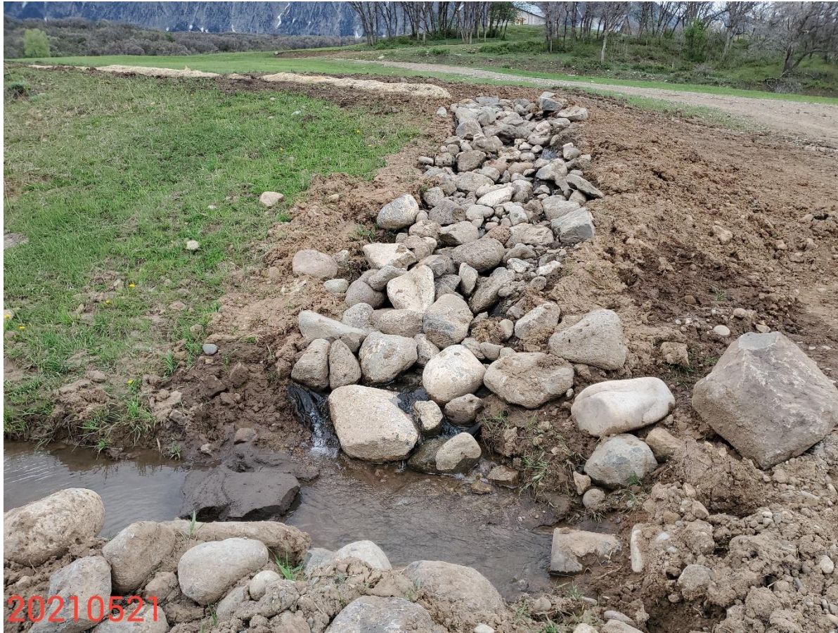
Photo 1: Photo taken from the east end of the Location, facing east. Photo shows section of the Location's perimeter stormwater diversion ditch armored with geotextile lining and rip-rap.
