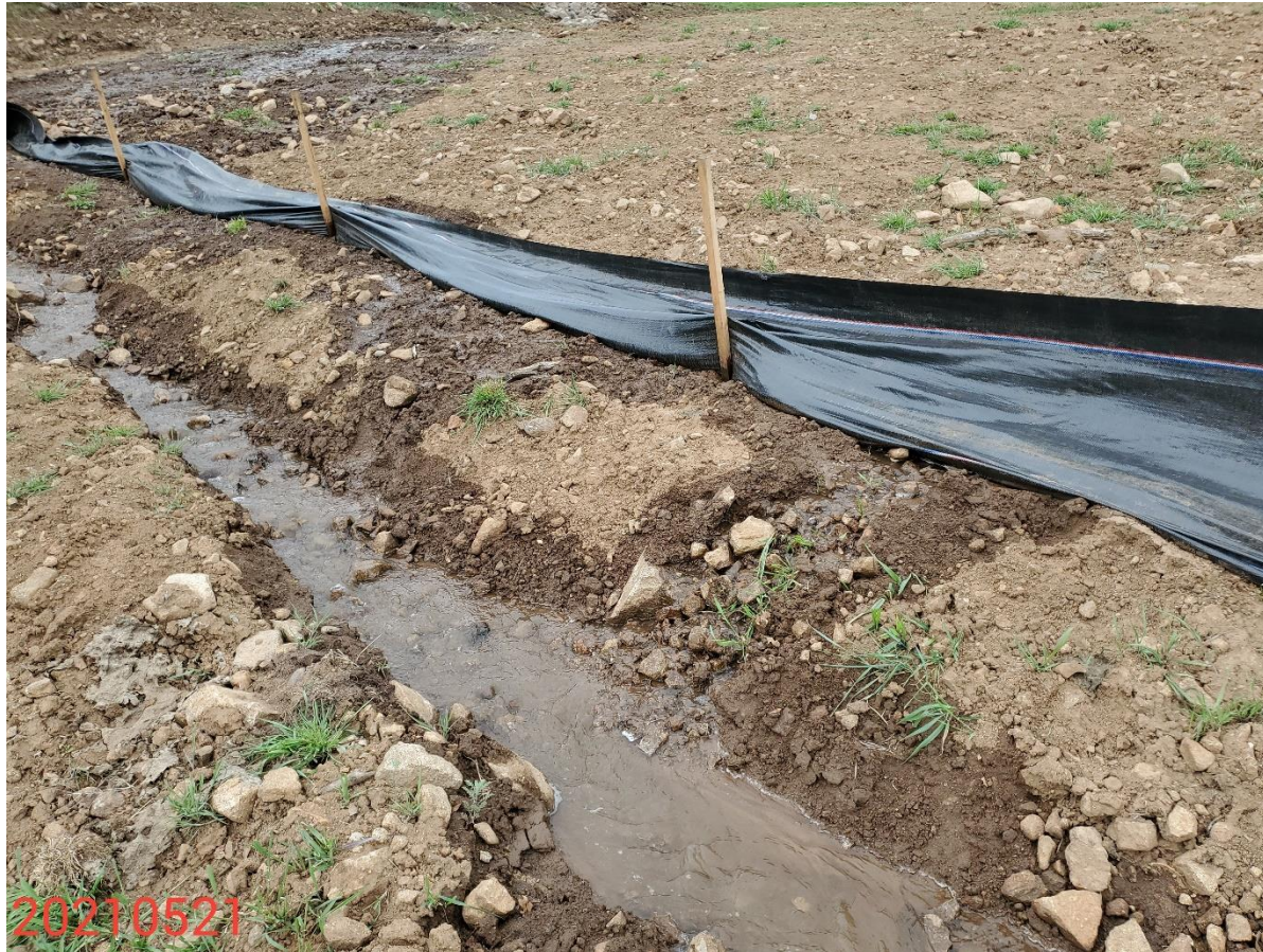
Photo 19: Photo shows silt fence along the western perimeter of the Location is inadequate and not in proper functioning condition.
