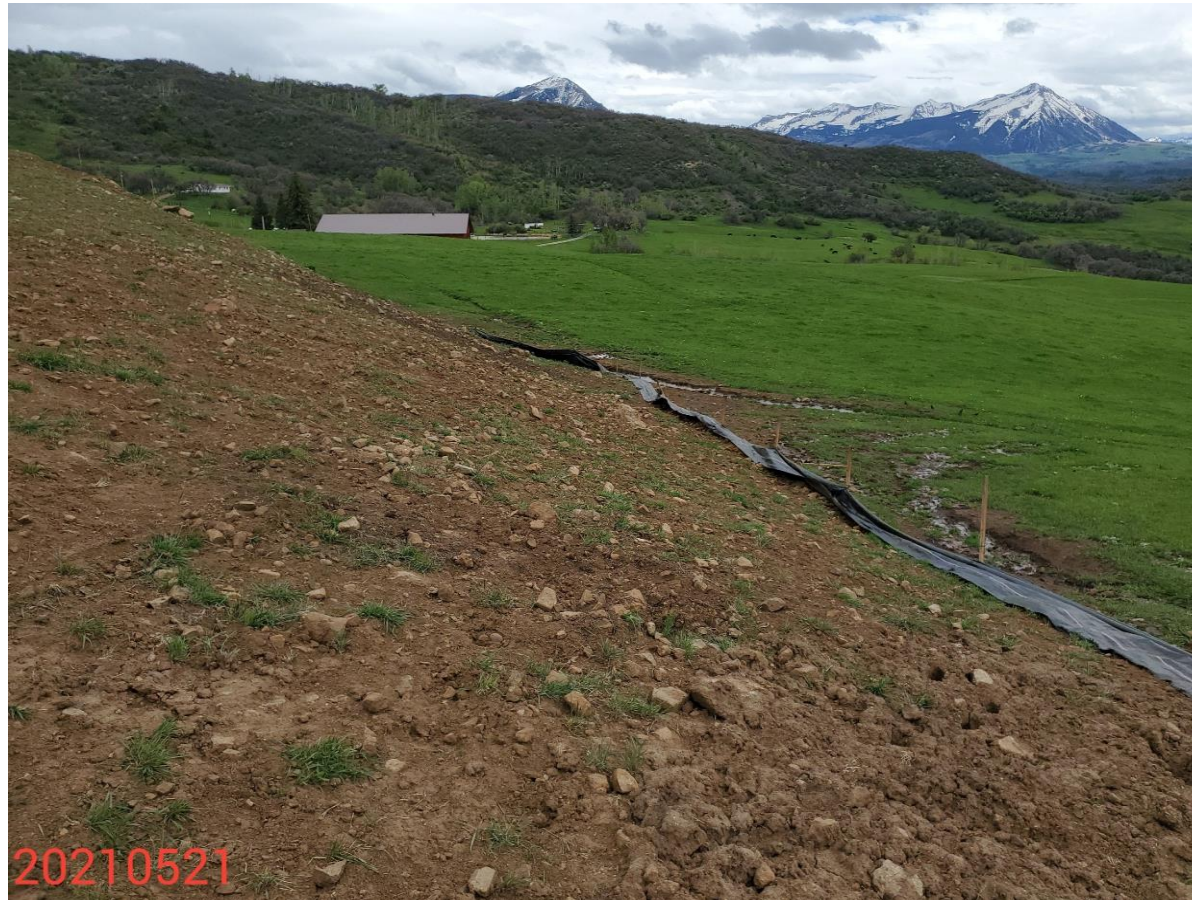
Photo 20: Photo shows silt fence along the western perimeter of the Location is inadequate and not in proper functioning condition.
