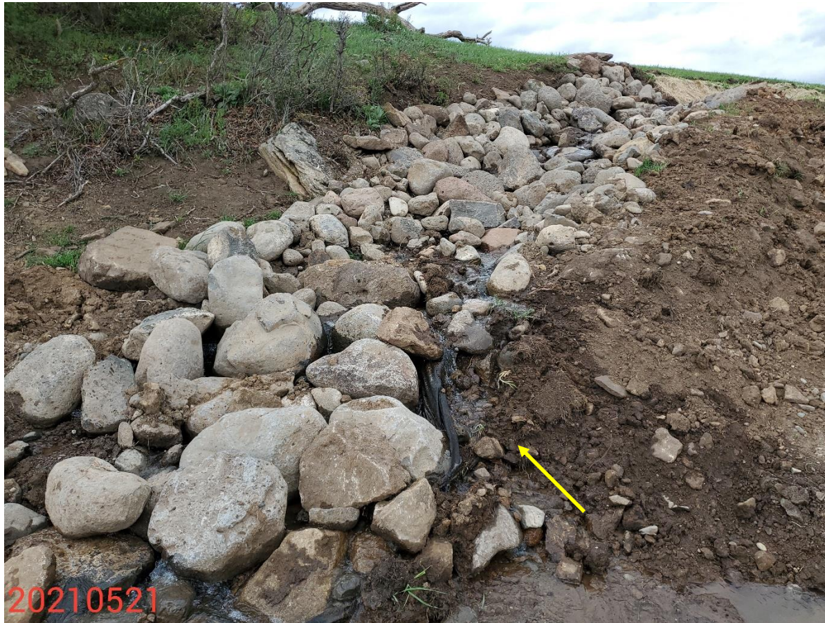
Photo 13: Photo taken from the northwest corner of the Location, facing north. Photo shows armored section of the Location's perimeter stormwater diversion; control measure inadequate/not in proper functioning condition; stormwater observed scouring/degrading around armor and geotextile lining.
