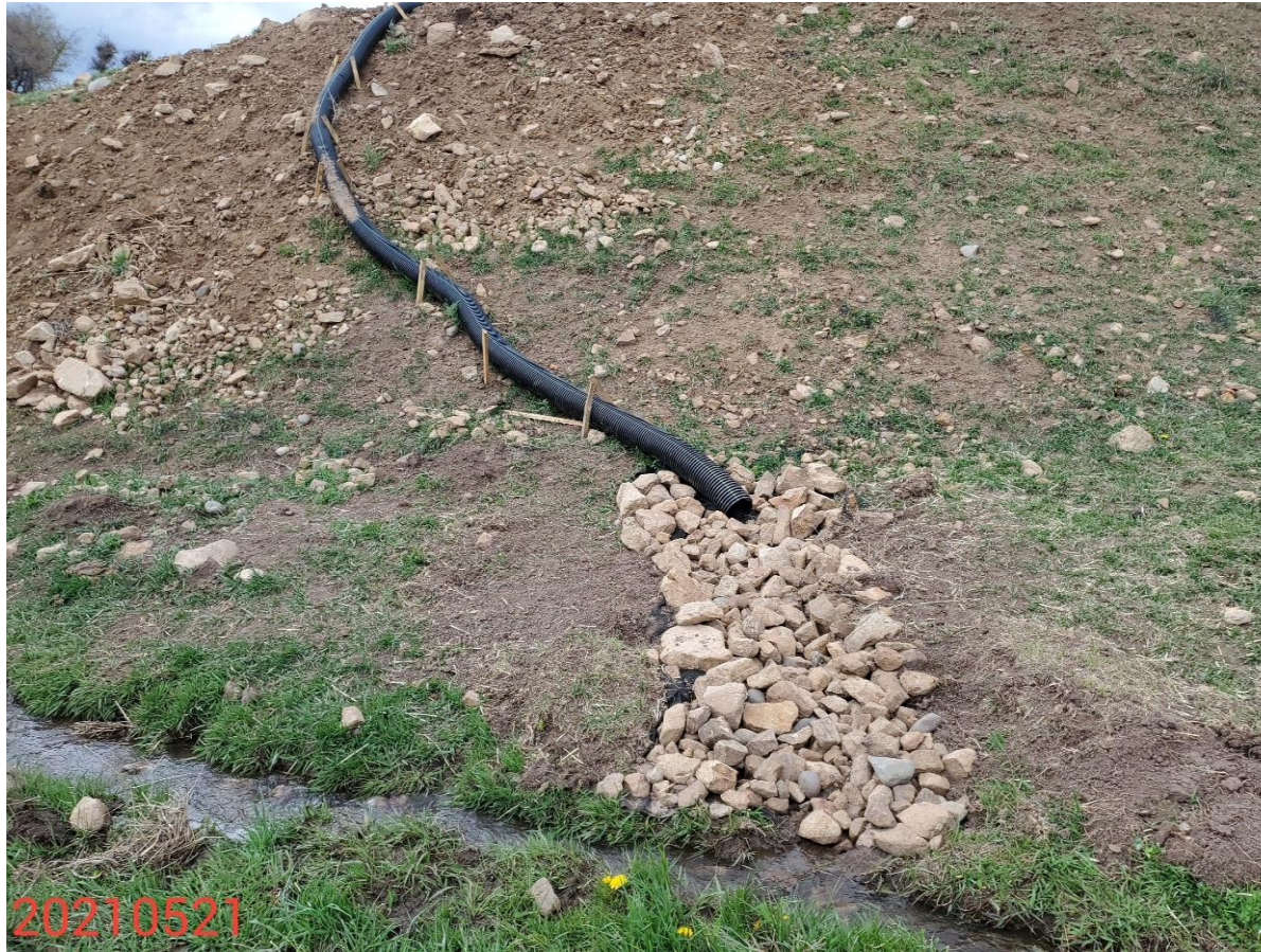
Photo 24: Photo taken from the southwest end of the Location, facing north. Photo shows slope drain; unclear if slope drain has been adequately secured. Outlet constructed with geotextile lining and rip-rap armor.
