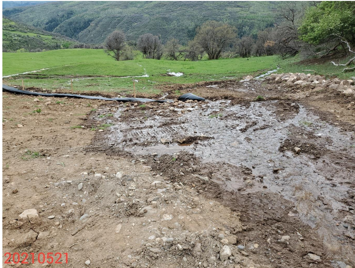
Photo 16: Continued from photo 15. Photo shows runoff from the ditch. Photo also shows silt fence along the western perimeter of the Location is inadequate and not in proper functioning condition.
