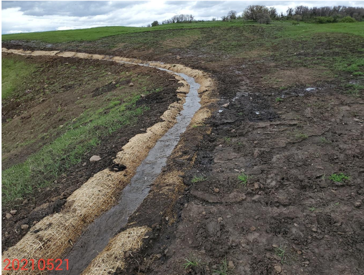
Photo 3: Photo taken from the east end of the Location, facing north. Photo shows the perimeter stormwater diversion ditch. Photo also shows control measures to protect/stabilize slopes and disturbed areas of the Location remain missing or insufficient. Unable to find evidence that revegetation activities were performed, and BMPs to stabilize seeded soils implemented. Erosion degradation evident.
