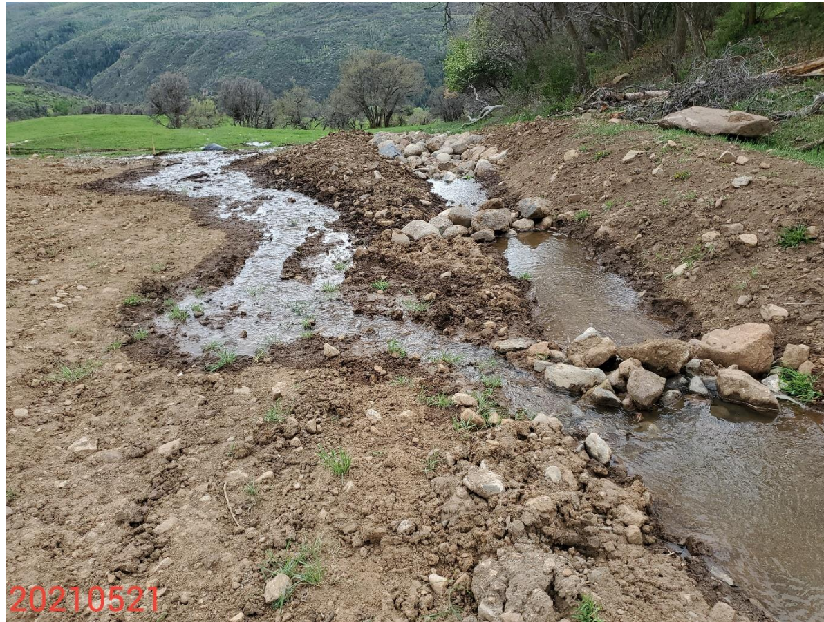
Photo 15: Photo taken from the stormwater diversion ditch on the northwest end of the Location, facing west. Photo shows perimeter stormwater diversion ditch installed on Location is inadequate/insufficient for the site's conditions; ditch not in proper functioning condition; stormwater has breached ditch resulting in additional stormwater erosion degradation.
