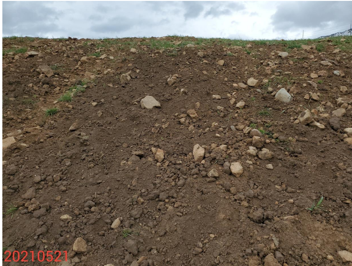
Photo 22: Photo taken from the slopes on the southwest end of the Location, facing north. Photo shows control measures to protect/stabilize slopes and disturbed areas of the Location remain missing or insufficient; unable to find evidence that revegetation activities were performed, and BMPs to stabilize seeded soils implemented.
