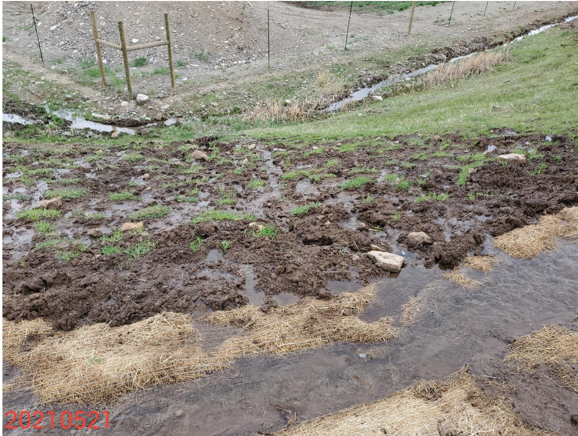
Photo 5: Continued from photo 4. Photo shows perimeter stormwater diversion ditch installed on Location is inadequate/insufficient for the site's conditions; ditch not in proper functioning condition. Photo also shows control measures to protect/stabilize slopes of the Location remain missing or insufficient.
