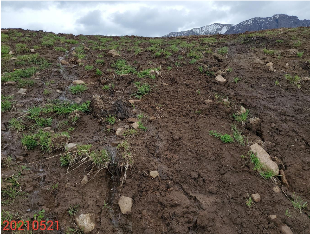
Photo 6: Continued from photo 5. Photo shows cut slopes on the Northeast end of the Location. Photo shows runon causing erosion degradation on the slopes. Control measures to protect/stabilize slopes and disturbed areas of the Location remain missing or insufficient. Unable to find evidence that revegetation activities were performed, and BMPs to stabilize seeded soils implemented.
