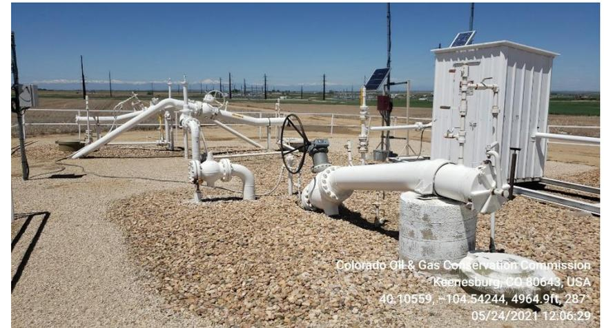
**Photo 5 Horizontal Heated Separator**
