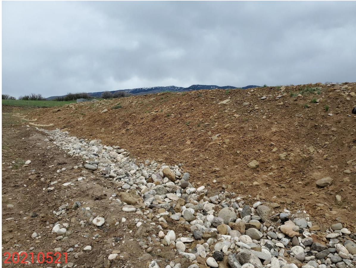
Photo 10: Photo taken from the slopes on the west end of the Location. Previous inspections documented that control measures to protect/stabilize slopes on the Location were missing or insufficient. Photo shows control measures to protect/stabilize slopes on the Location remain missing or insufficient.
