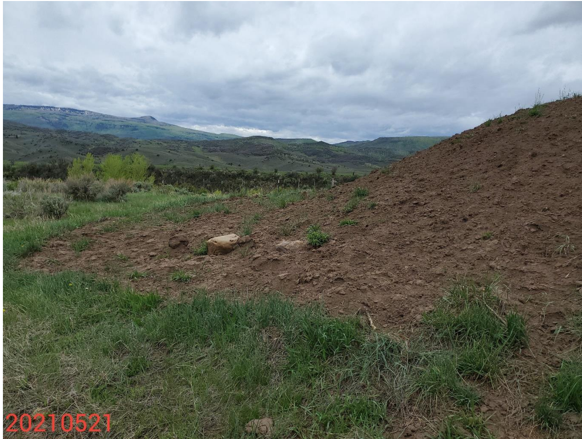
Photo 13: Photo taken from the topsoil stockpile on the west end of the Location. Previous inspections documented that control measures to protect/stabilize slopes on the Location were missing or insufficient. Photo shows control measures to protect/stabilize slopes on the Location remain missing or insufficient.
