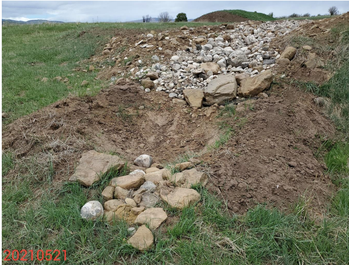
Photo 8: Photo taken from the southwest corner of the Location. Photo shows sediment trap. Precious inspections documented that the sediment trap has not been constructed with an appropriate outlet per good engineering practices. Photo shows outlet has not been not constructed in accordance with good engineering practices; outlet missing geotextile lining; scouring/degradation becoming evident around riprap at outlet. Trap also does not appear to be appropriate in size.
