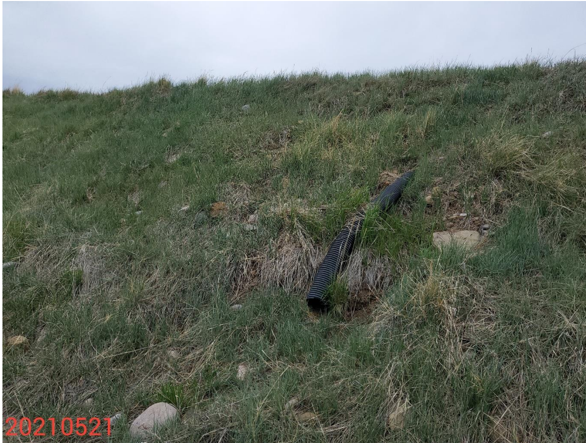
Photo 5: Photo taken from the southeast corner of the Location. Photo shows slope drain. Previous inspections documented that the slope drain was not constructed with an appropriate outlet per good engineering practices. Photo shows slope drain has not been constructed with an appropriate outlet.
