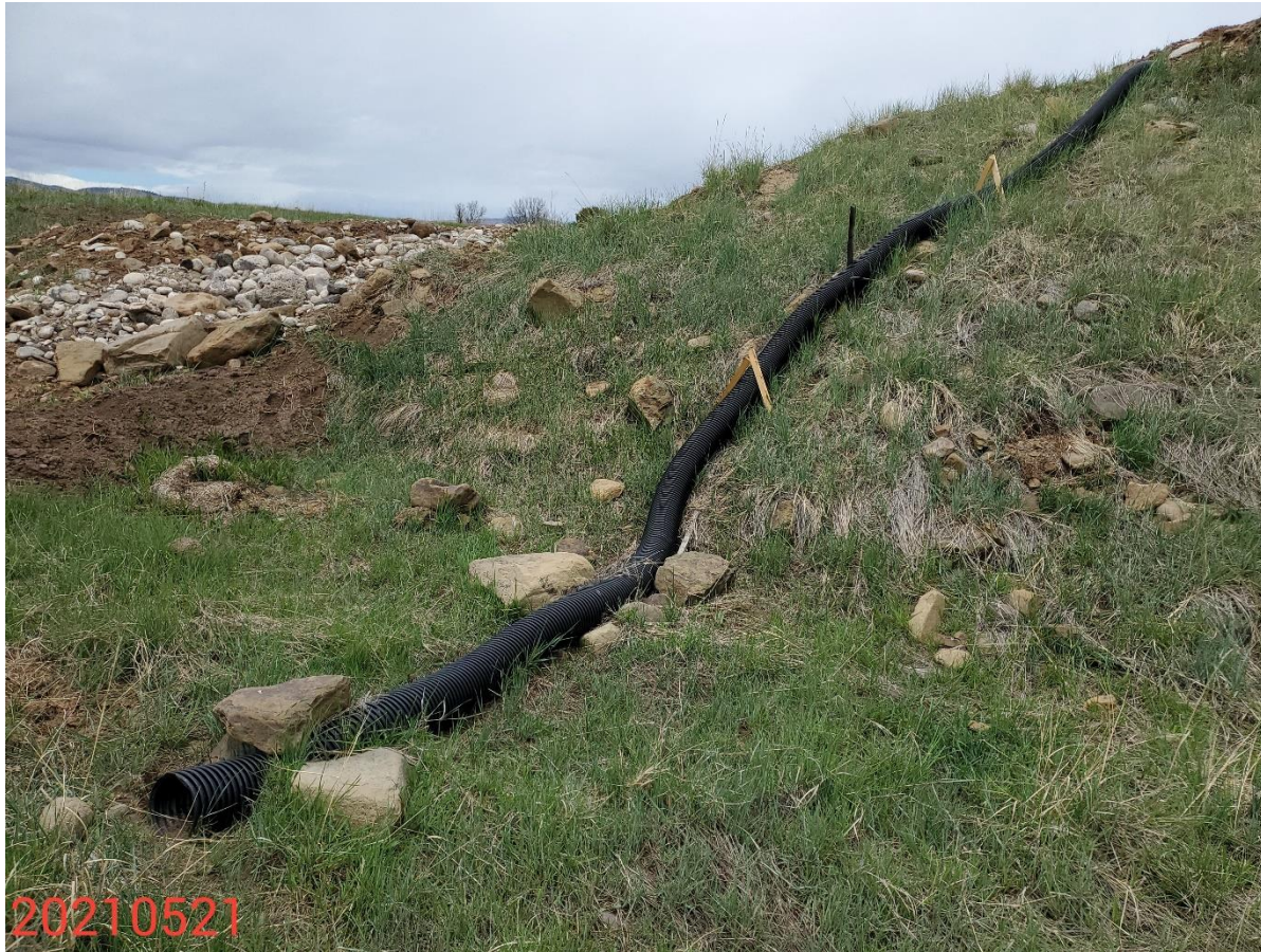
Photo 6: Photo taken from the southwest corner of the Location. Photo shows slope drain. Previous inspections documented that the slope drain has not been constructed with an appropriate outlet per good engineering practices. Photo shows slope drain remains improperly constructed with an appropriate outlet per good engineering practices.
