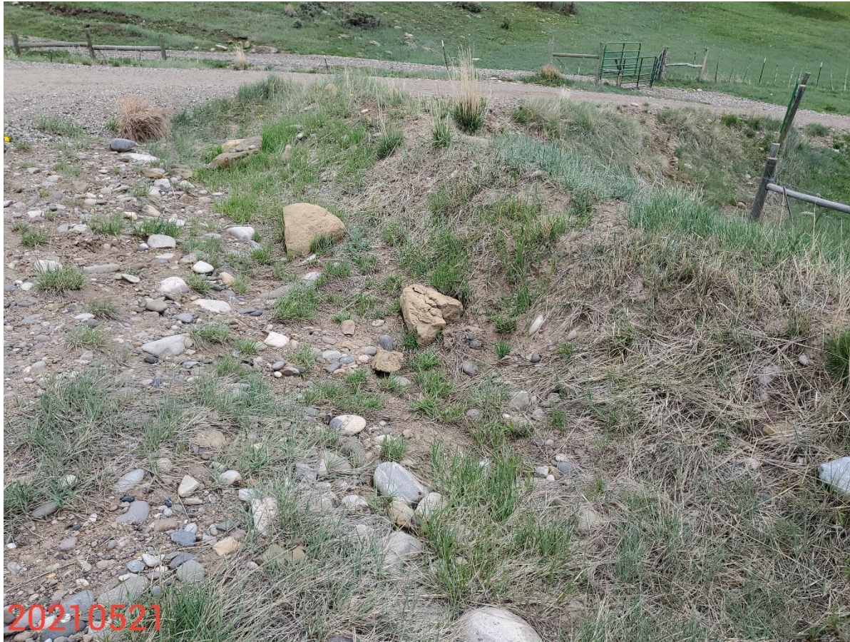
Photo 4: Photo taken from the southeast corner of the Location. Previous inspections observed that the Slope drone has not been maintained in proper functioning condition; inlet filled with sediment. Photo shows inlet of the slope drain remains filled with sediment.
