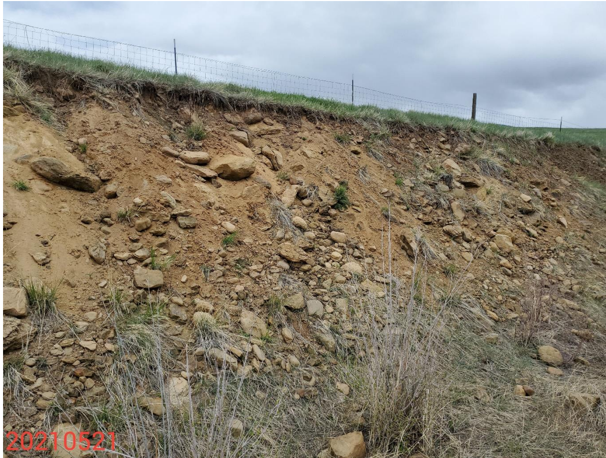
Photo 16: Photo taken from the north end of the Location. Previous inspections documented that control measures to protect/stabilize slopes on the Location were missing or insufficient. Photo shows control measures to protect/stabilize slopes on the Location remain missing or insufficient.
