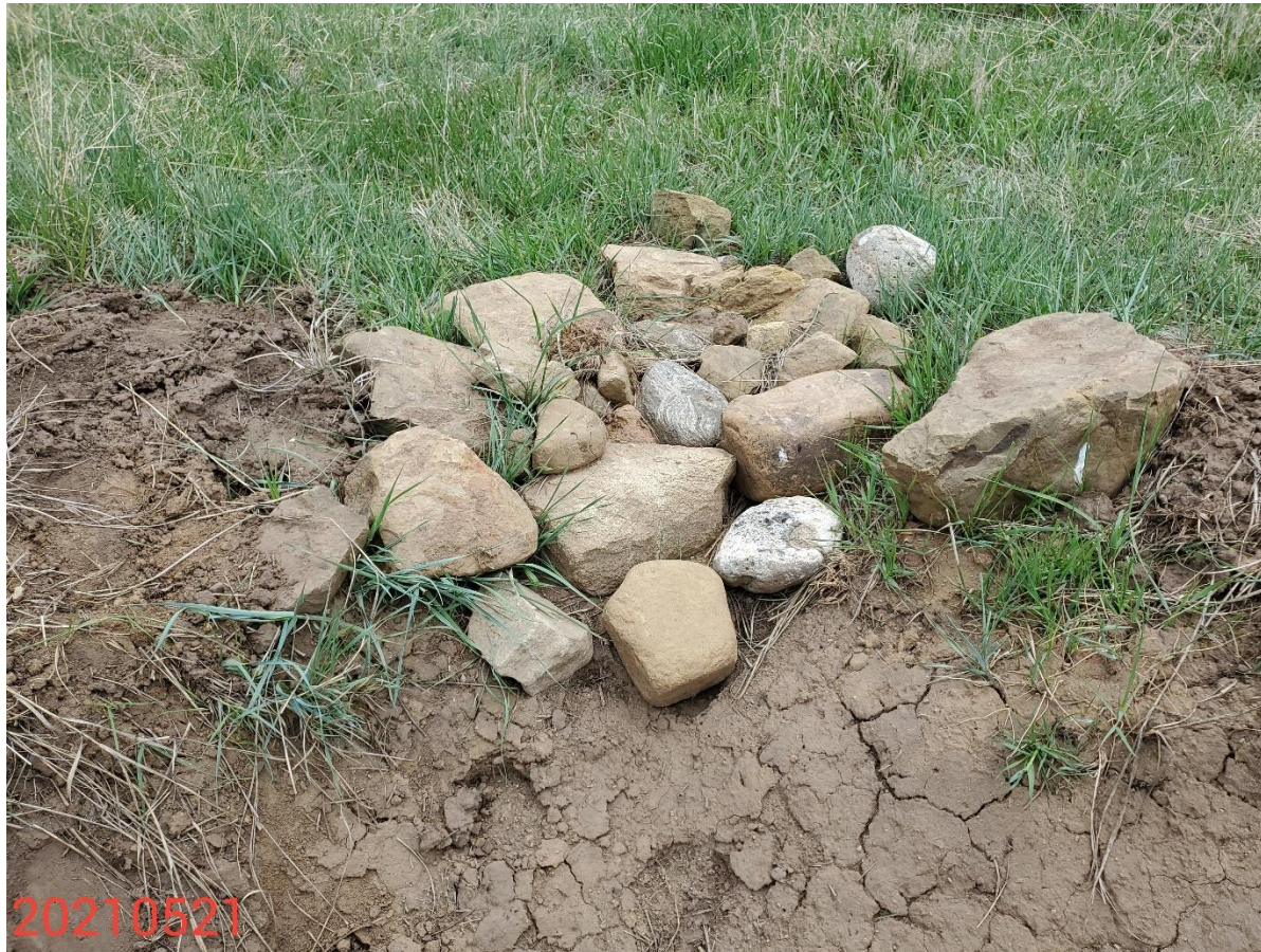
Photo 9: See comments under photo 8. Photo shows outlet missing geotextile lining per good engineering practices; scouring/degradation becoming evident around riprap at outlet
