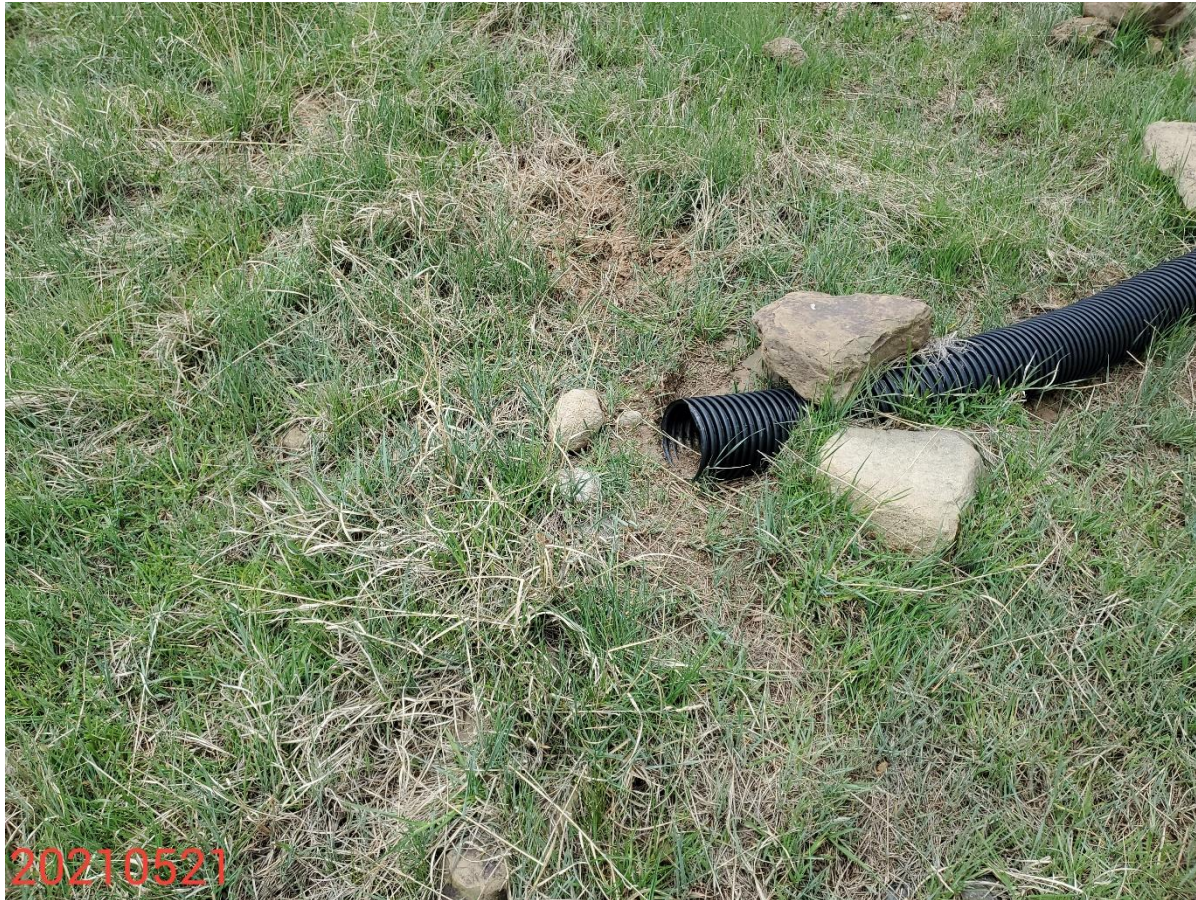
Photo 7: Continued from photo 6. Photo shows slope drain has not constructed with an appropriate outlet per good engineering practices.
