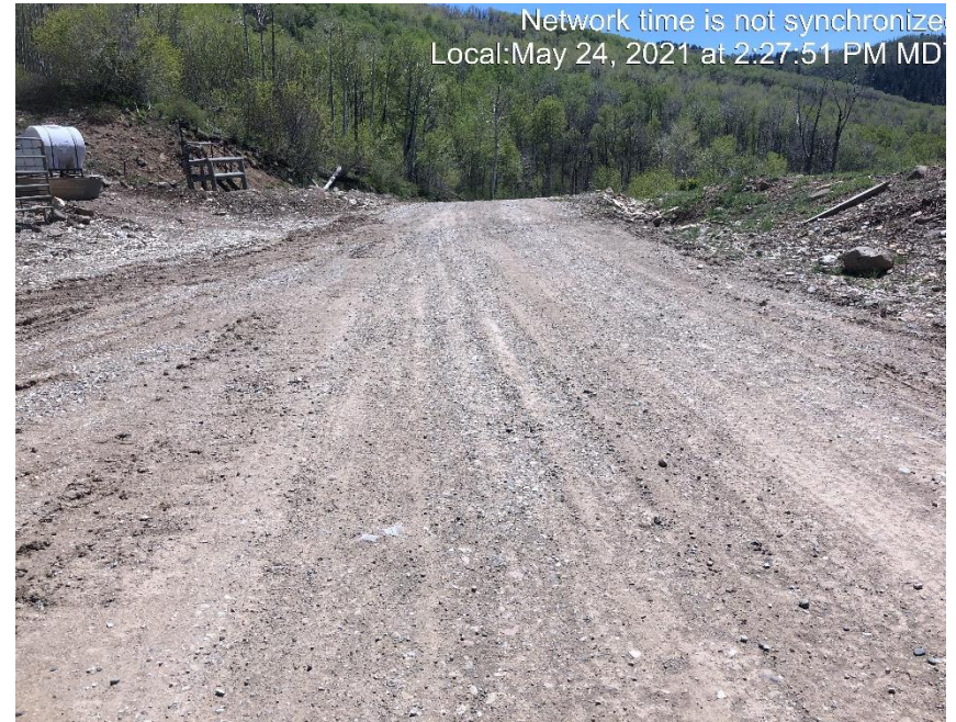
Photo #3922 No form of tracking BMP located at entrance to location.
