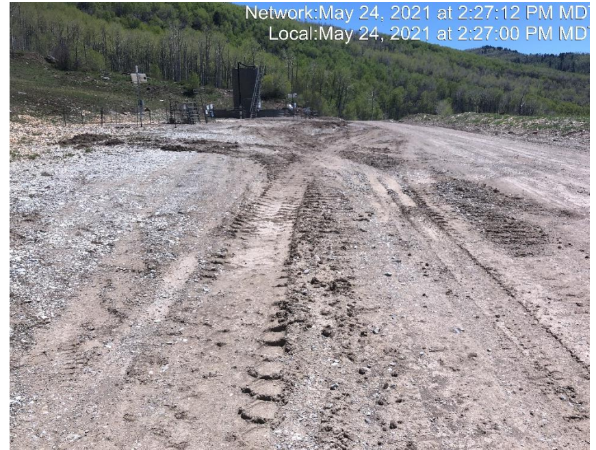
Photo #3920 Location lacks stabilization.
