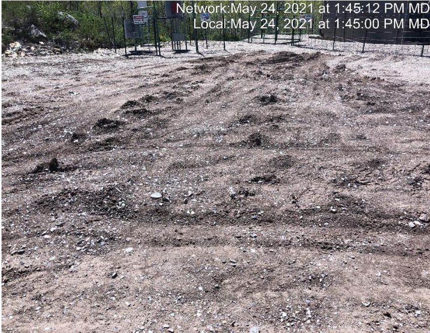
Photo #3918 Location lacks stabilization.
