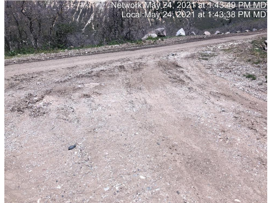
Photo #3915 No form of tacking BMP located at entrance to location.
