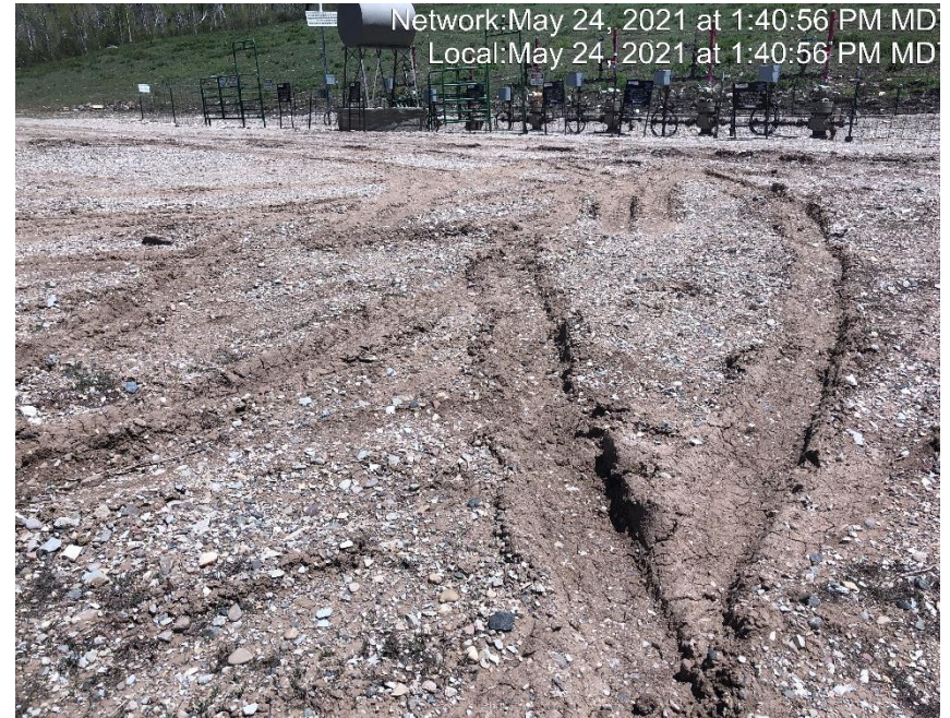
Photo #3914 Location lacks stabilization.
