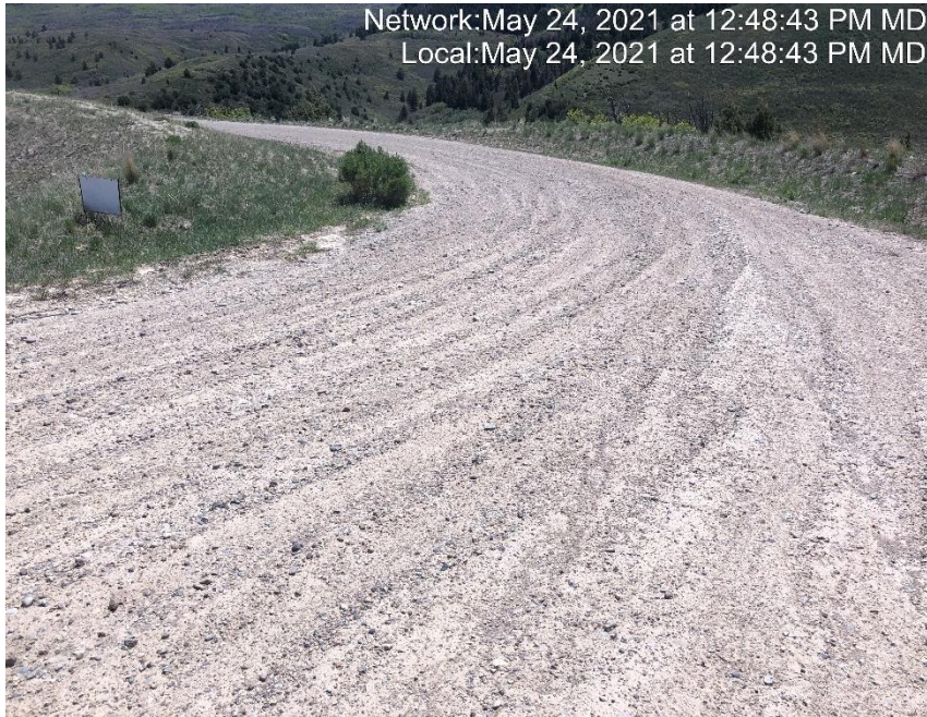
Photo #3908 No form of tracking BMP located at the entrance to location.
