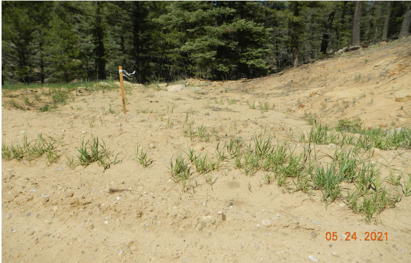
Photo 2. There is a sediment trap along the access road that is filled in with sediment.
