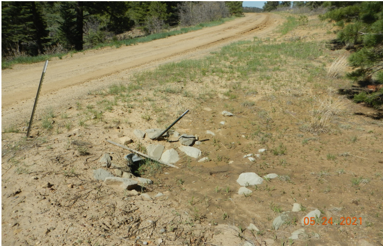
Photo 3. This culvert is partially filled in with sediment at Lat/Long:37.2112, - 104.9298.
