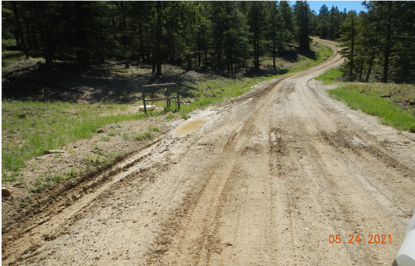
Photo 4. Stormwater is not properly directed toward the culvert and there is gravel obstructing the culvert.
