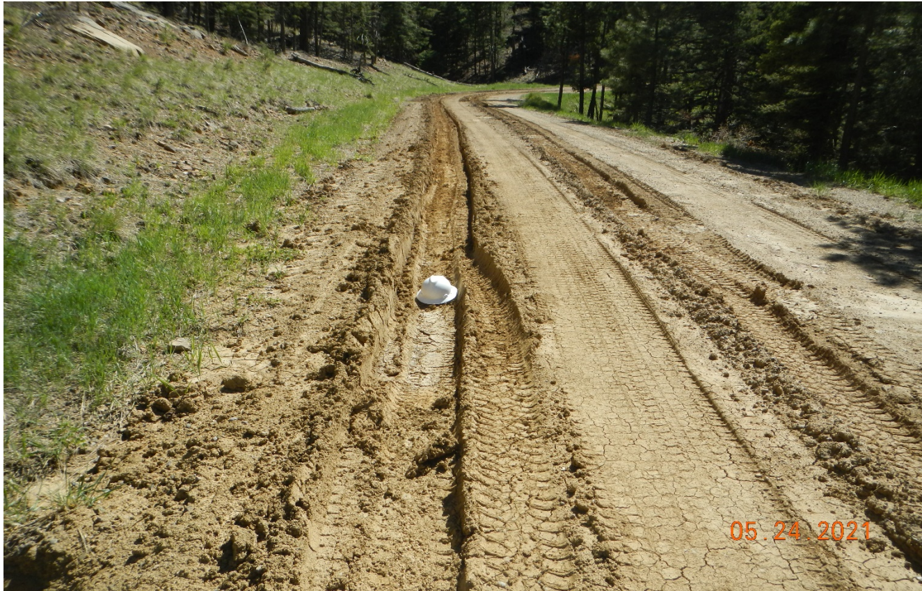
Photo 7. Facing west along the main access road. There are areas along the road that have vehicle rutting and erosion. The road needs to be maintained and stabilized.
