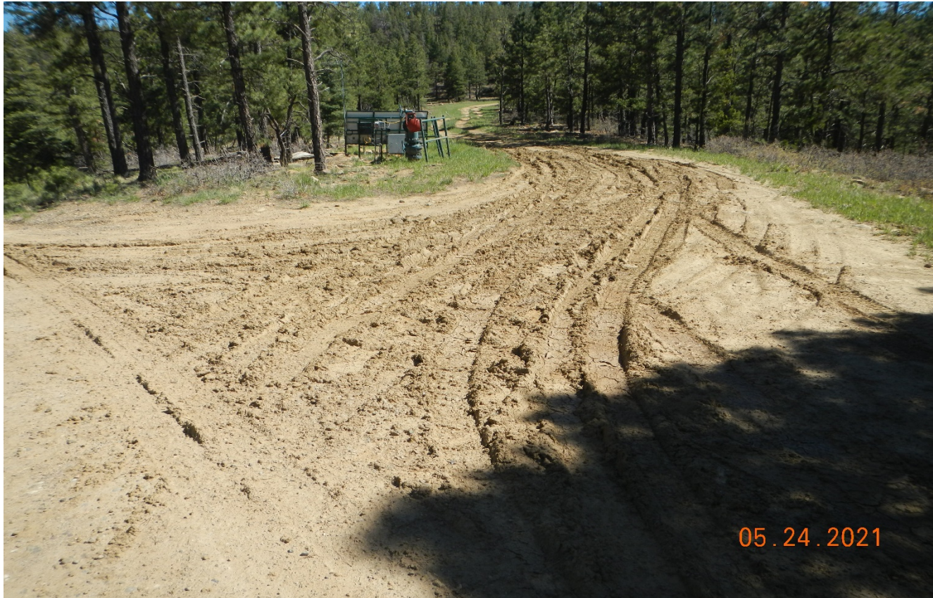
Photo 8. There is vehicle rutting where trucks are backing into the receiver/launcher.
