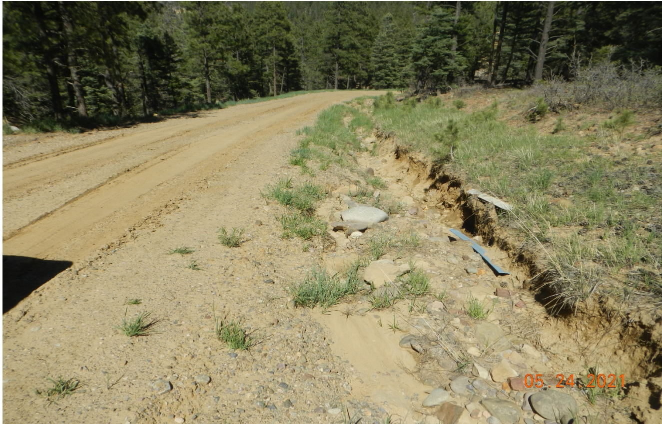
Photo 6. BMP's need to be installed along the side of the road to prevent erosion at this area, Lat/Long:37.20905,-104.9369.
