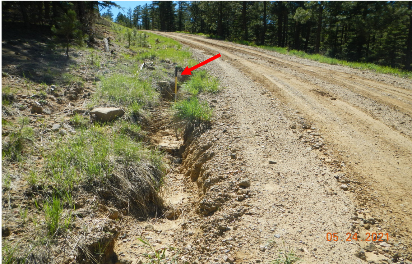
Photo 5. There is an erosion channel along the side of the road. Arrow points to 4.5 ft. shovel to show depth of erosion.
