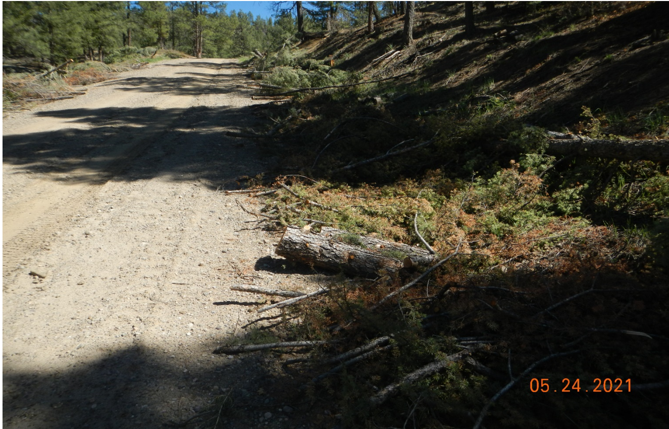
Photo 1. It was observed that branches and logs are being piled along the side of the road. It is a concern that braches and logs will obstruct stormwater flow and direct stormwater onto the road.
