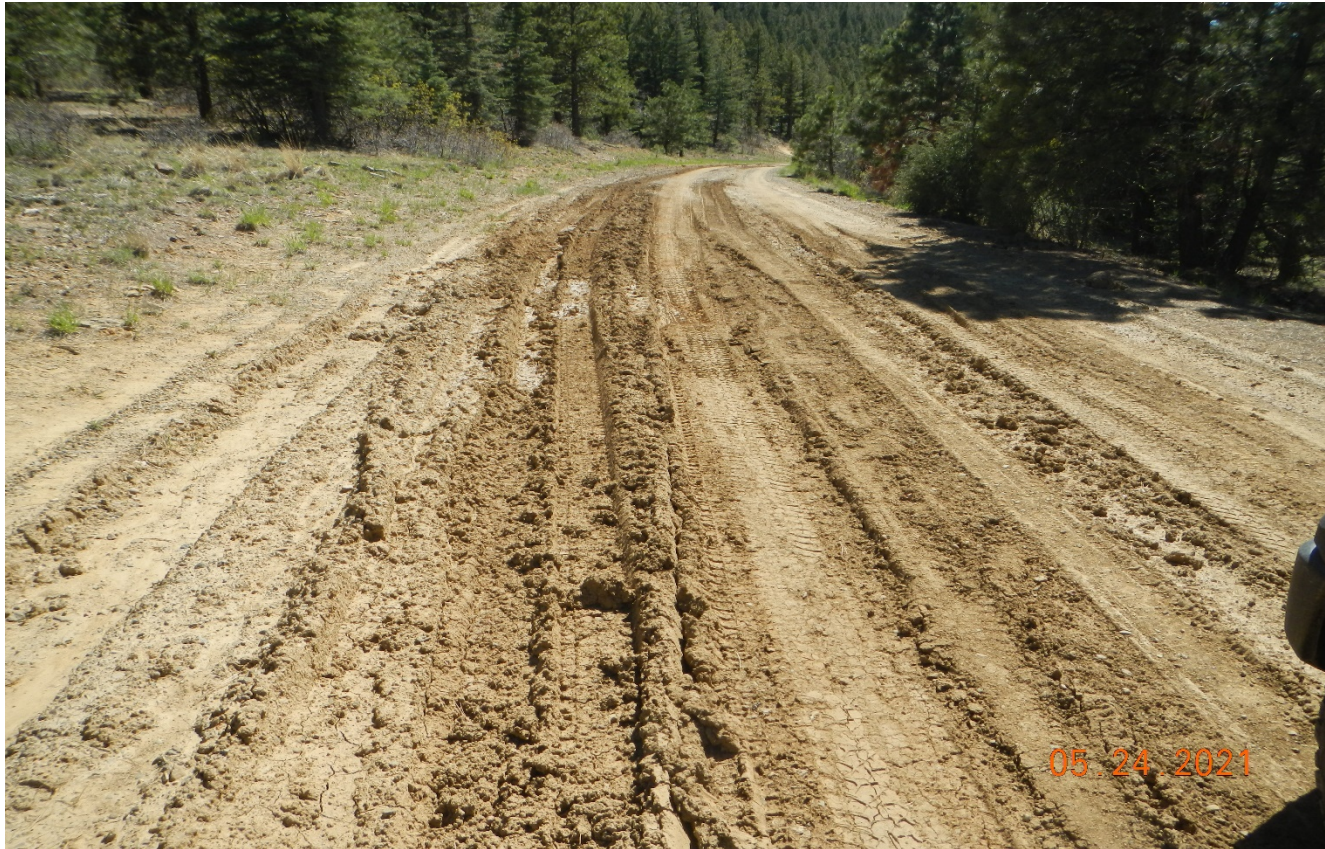
Photo 2. Facing west along the main access road. There are areas along the road that have vehicle rutting and erosion.
