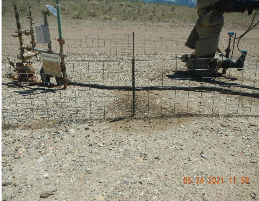
Stained ground around injection well head.
