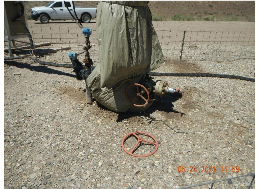
Stained ground around injection well head.
