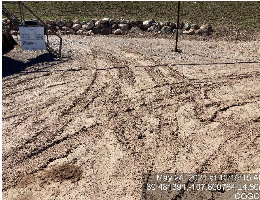
Lack of stabilization/compaction
