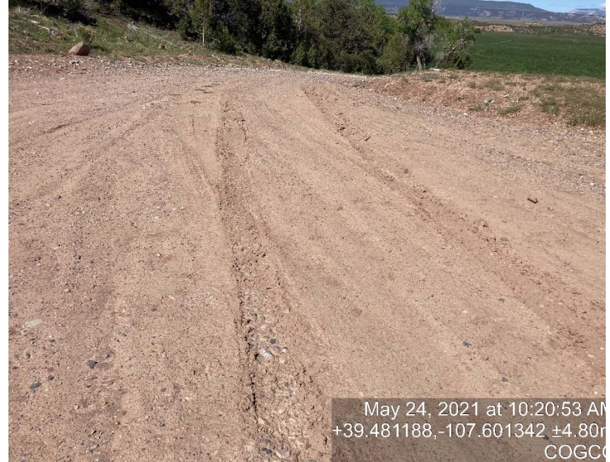
Lack of stabilization/compaction looking South/west leaving pad
