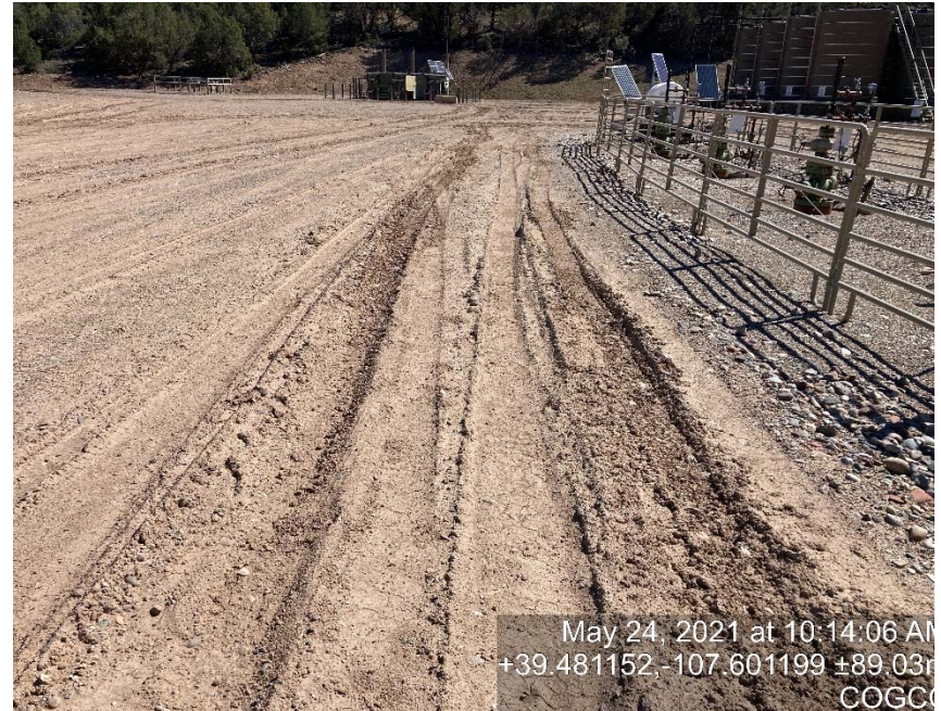
Lack of stabilization/compaction
