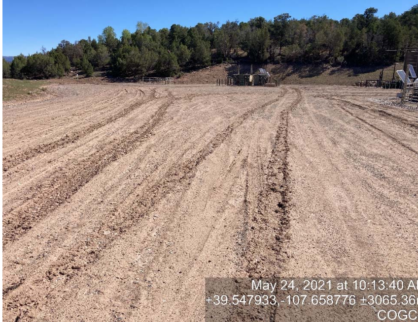
Lack of stabilization/compaction looking north into pad
