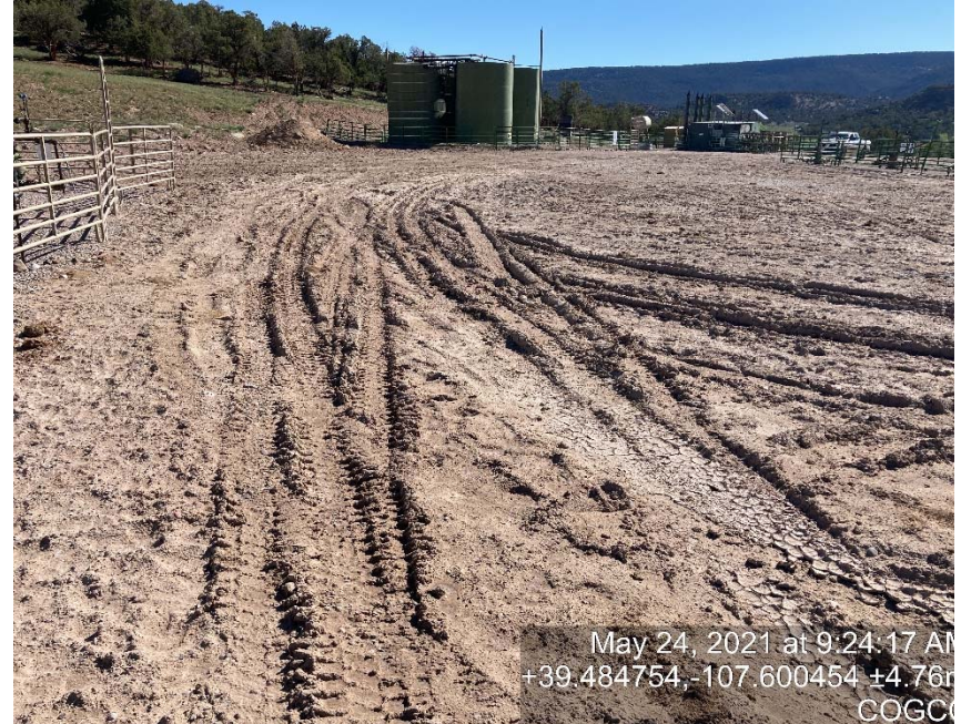
Lack of stabilization/compaction
