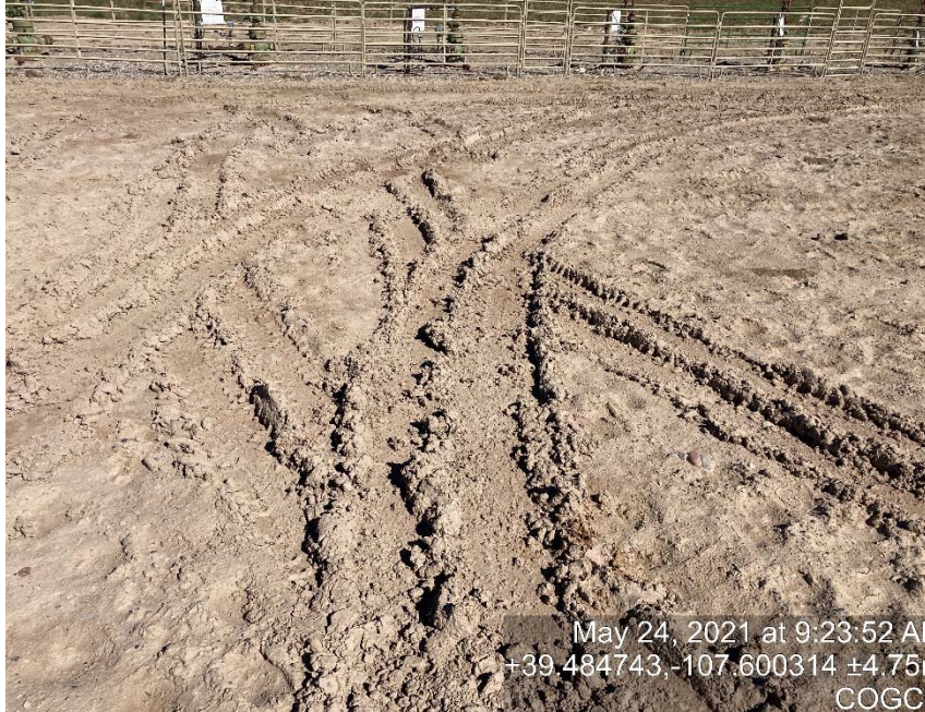
Lack of stabilization/compaction
