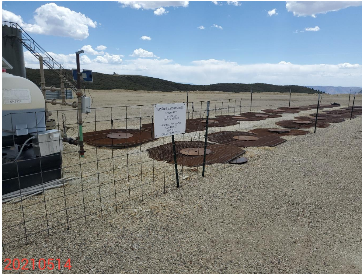
Photo 4: Photo taken from the wells. Permits for undrilled wells on the Location have been deleted. Photo shows conductor settings/cellars require closure and reclamation in accordance with Rule 406.e.
