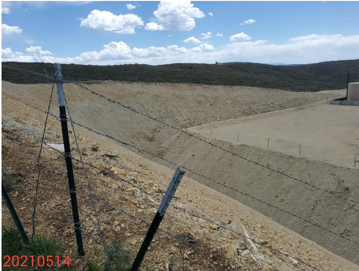
Photo 1: Photo taken from the north end of the Location, facing southeast. Photos 1-3 provide an overview of the Location from southeast, south to southwest. Photos show interim reclamation of the Location has not been conducted in accordance with 1003 rules.
