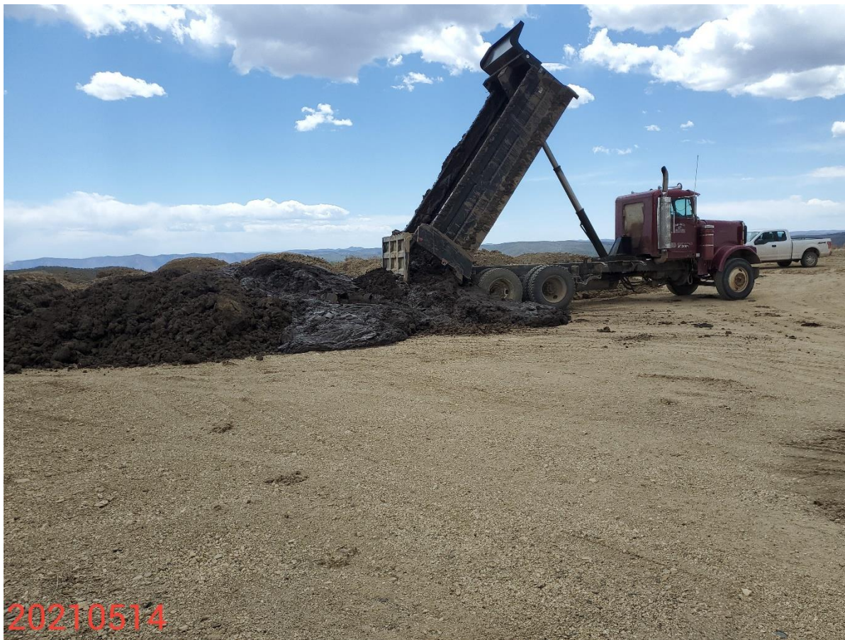
Photo 7: Photo taken from the southeast end of the Location. Photo shows a Operator in process of hauling material from sediment traps in the Crystal Creek area, and placing /storing on the Location. Operator stated in an email that TEP have “historically used sediment trap clean out materials to supplement top soil for any reclaims that may be going on in the local area”.
