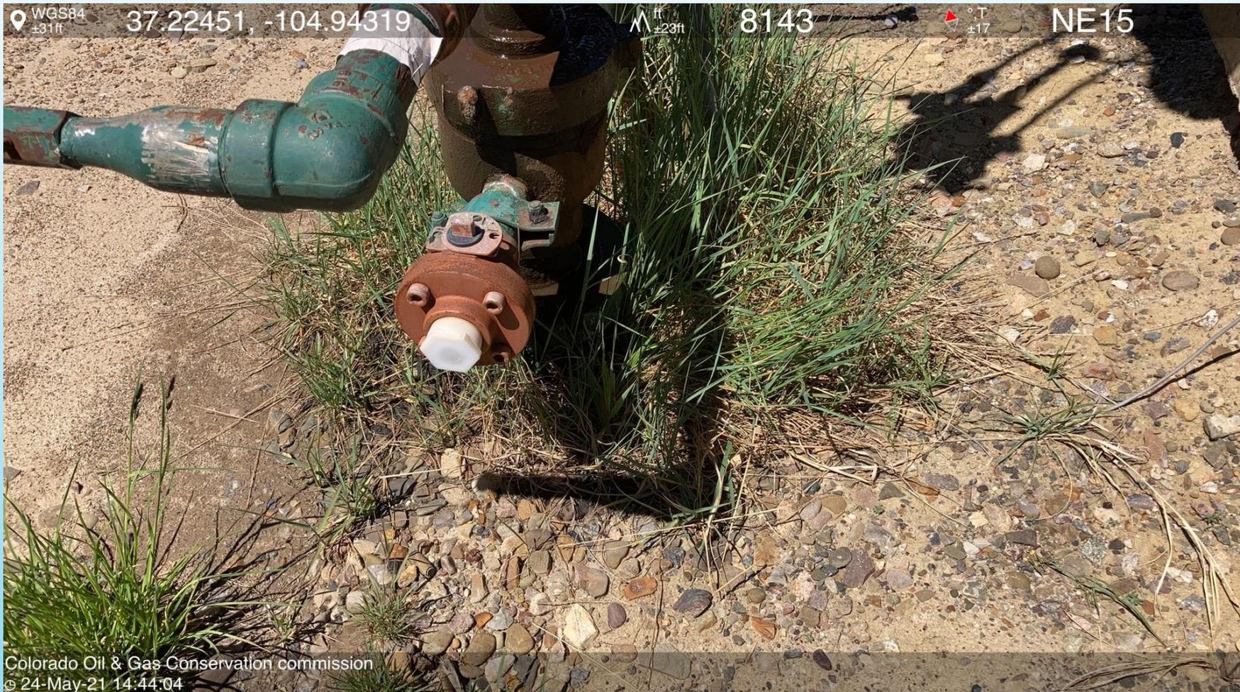
**PHOTO 3: Bradenhead inaccessible or not visible on original well. Install appropriate fittings to allow bradenhead visual inspection as per Rule 419.a.(1), (2) CA DATE 6-7-21.**
