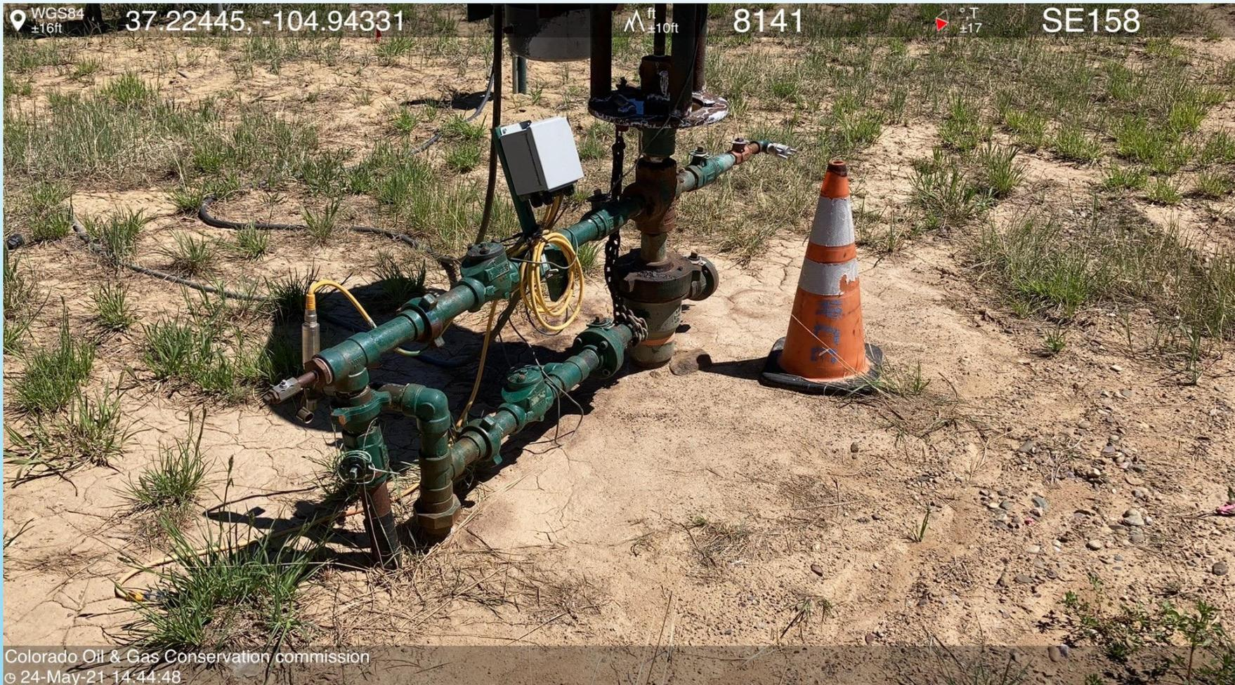
**PHOTO 4: Bradenhead inaccessible or not visible on TR well. Install appropriate fittings to allow bradenhead visual inspection as per Rule 419.a.(1), (2) CA DATE 6-7-21.**
