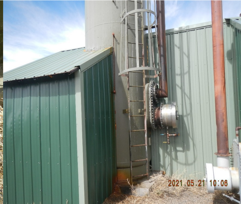
Staining of soil, concrete pad, and building from apparent leak. Note: weeds.
