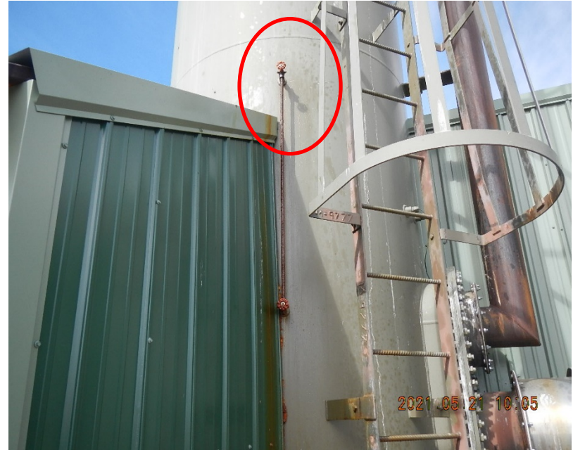
Apparent leak near a valve on the separator.
