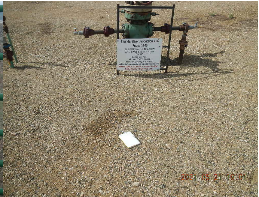
Wellhead sign. Note incorrect operator information. And staining in front of and behind well.
