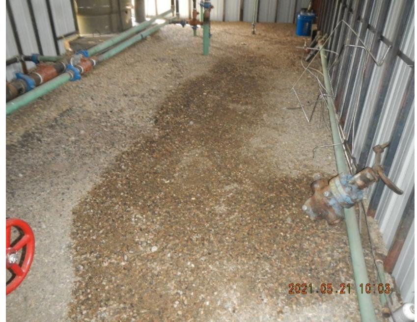
Soil staining within treater building.
