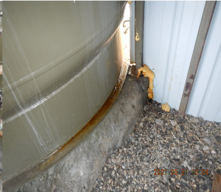
Condensate from apparent valve leak,
