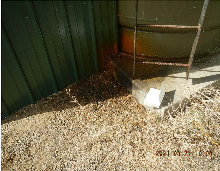
Staining of soil, concrete pad, and building from apparent leak.
