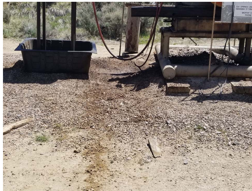
Photo 3. Stained soil at pump jack.
