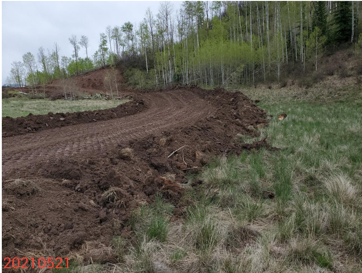
Photo 10: Photo taken from the newly constructed access road south of the Location, facing northeast. Photo shows stormwater and erosion control measures along the access road are missing or insufficient.
