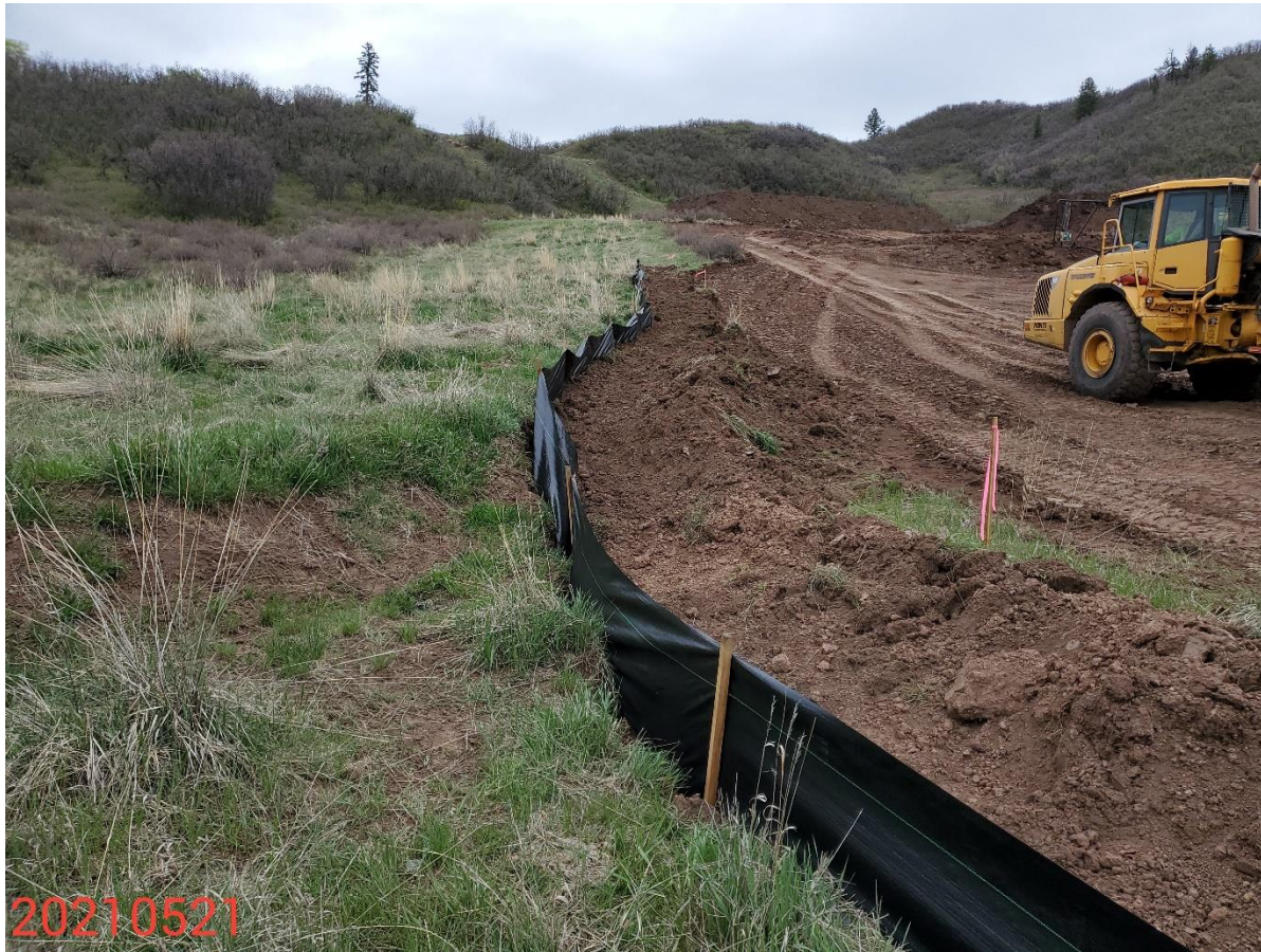
Photo 4: Photo shows silt fence constructed along the southern and western perimeters of the Location.
