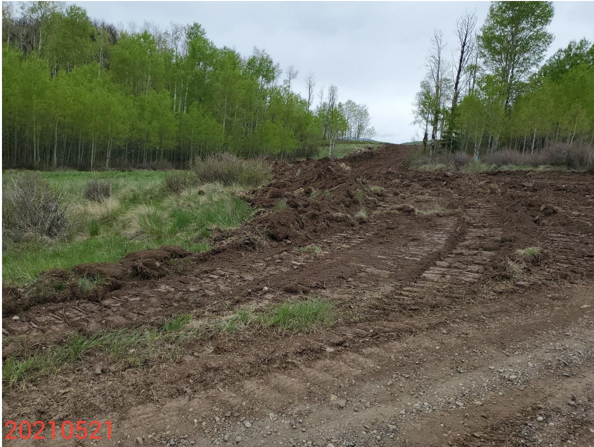
Photo 11: Photo taken from the newly constructed access road east of the Location, facing southwest. Photo shows stormwater and erosion control measures along the access road are missing or insufficient.
