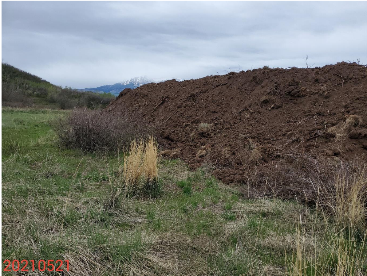
Photo 5: Photo taken from the topsoil stockpile on the north end of the Location. Photo shows stormwater BMPs at the soil stockpile to prevent offsite sediment transport are missing or insufficient.
