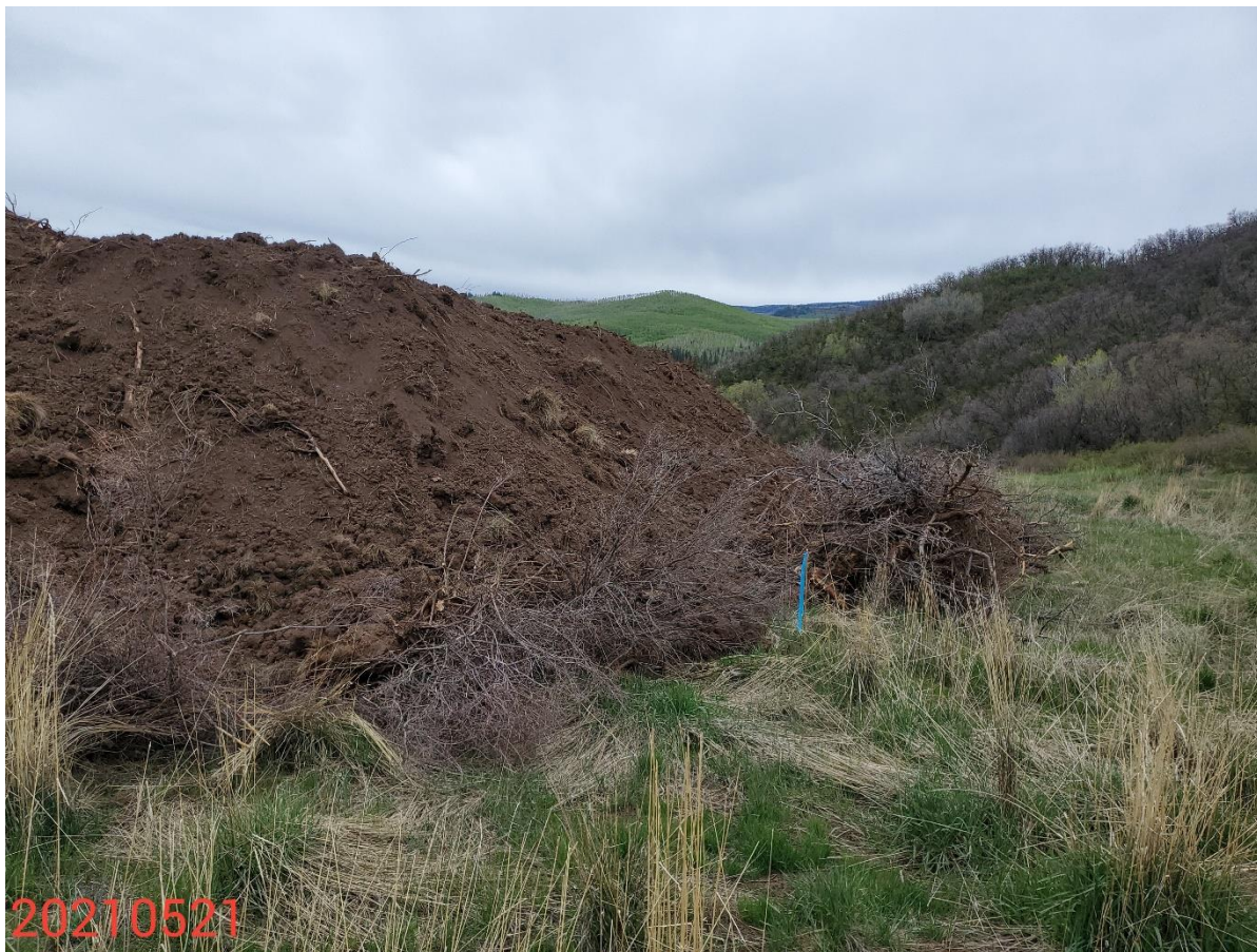
Photo 6: Photo taken from the topsoil stockpile on the north end of the Location. Photo shows stormwater BMPs at the soil stockpile to prevent offsite sediment transport are missing or insufficient.
