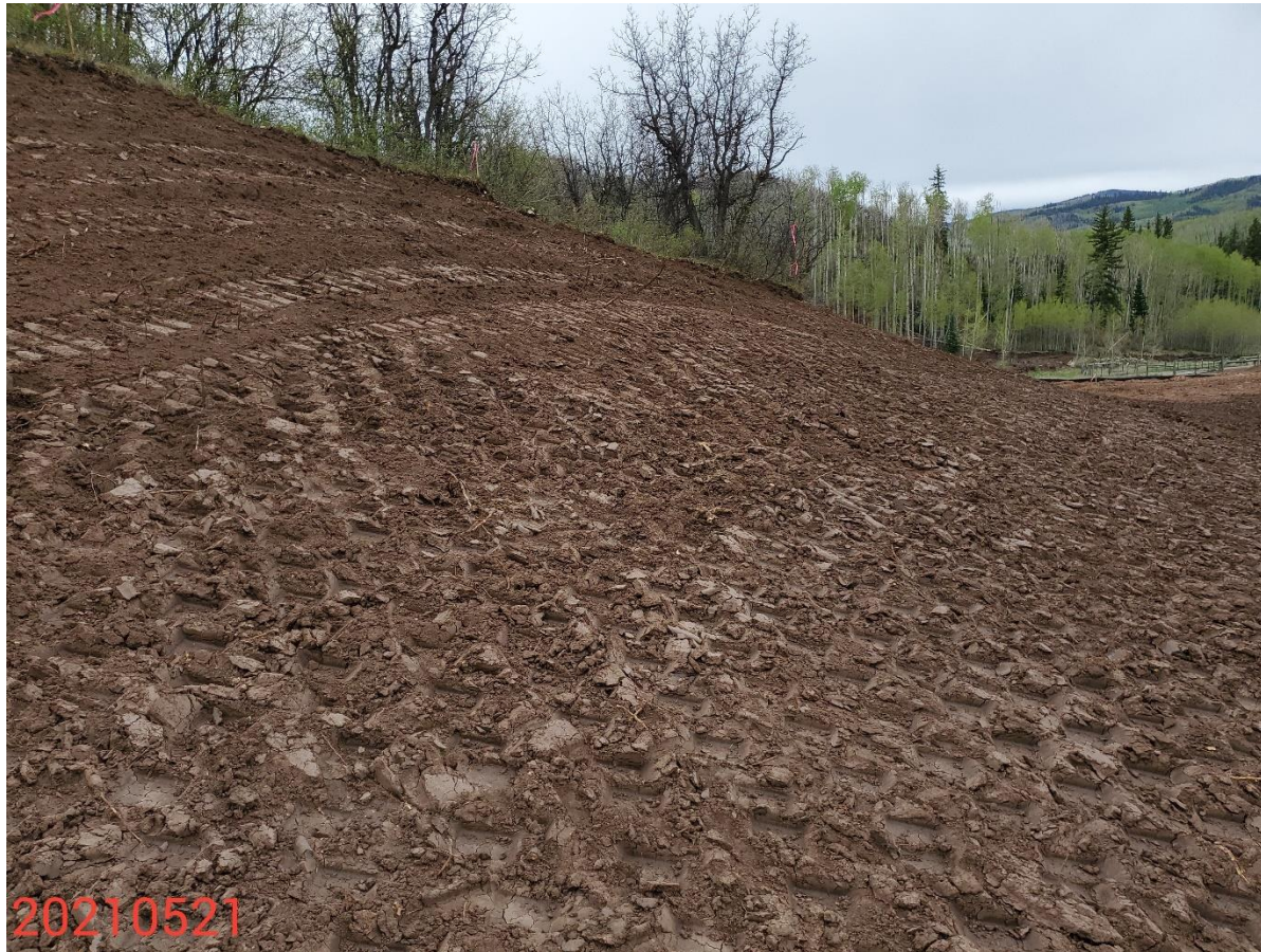
Photo 9: Photo of the cut slope on the east end of the cut slope. Photo shows surface roughening to stabilize soils on the slope.
