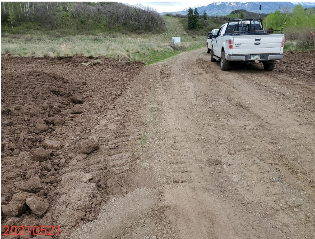
Photo 2: Photo taken from the east end of the Location, facing southeast. Photo shows Location entrance. Though off-site sediment transport concerns were not observed, photo shows that control measures to prevent vehicle sediment tracking are missing. Advise implementing control measures to mitigate/minimize off-site sediment transport prior to tracking issues.
