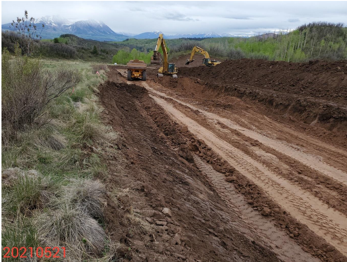
Photo 7: Photo taken from the north end of the Location, facing southeast. Photo shows location construction, and soil salvage/segregation activities in process.
