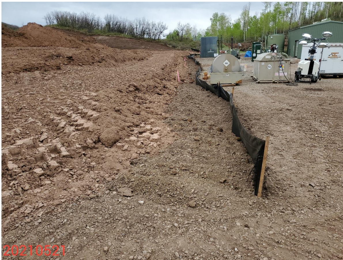
Photo 3: Photo shows silt fence constructed along the southern and western perimeters of the Location.
