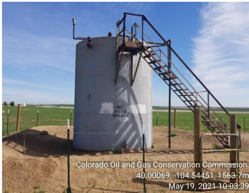
Photo 3 crude oil tank no markings or placards. Tank not painted.
