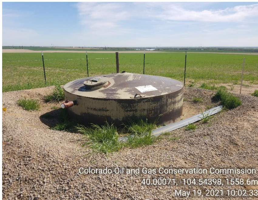
Photo 1 Production Tank not markings or placards. Tank not painted
