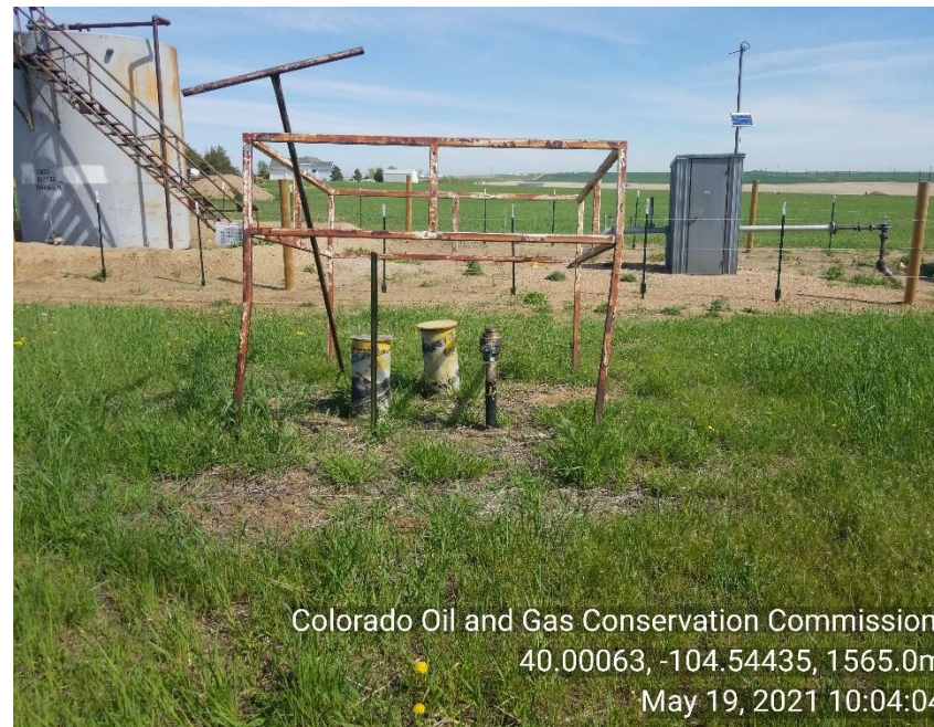
Photo 4 unmarked not LOTO risers.
