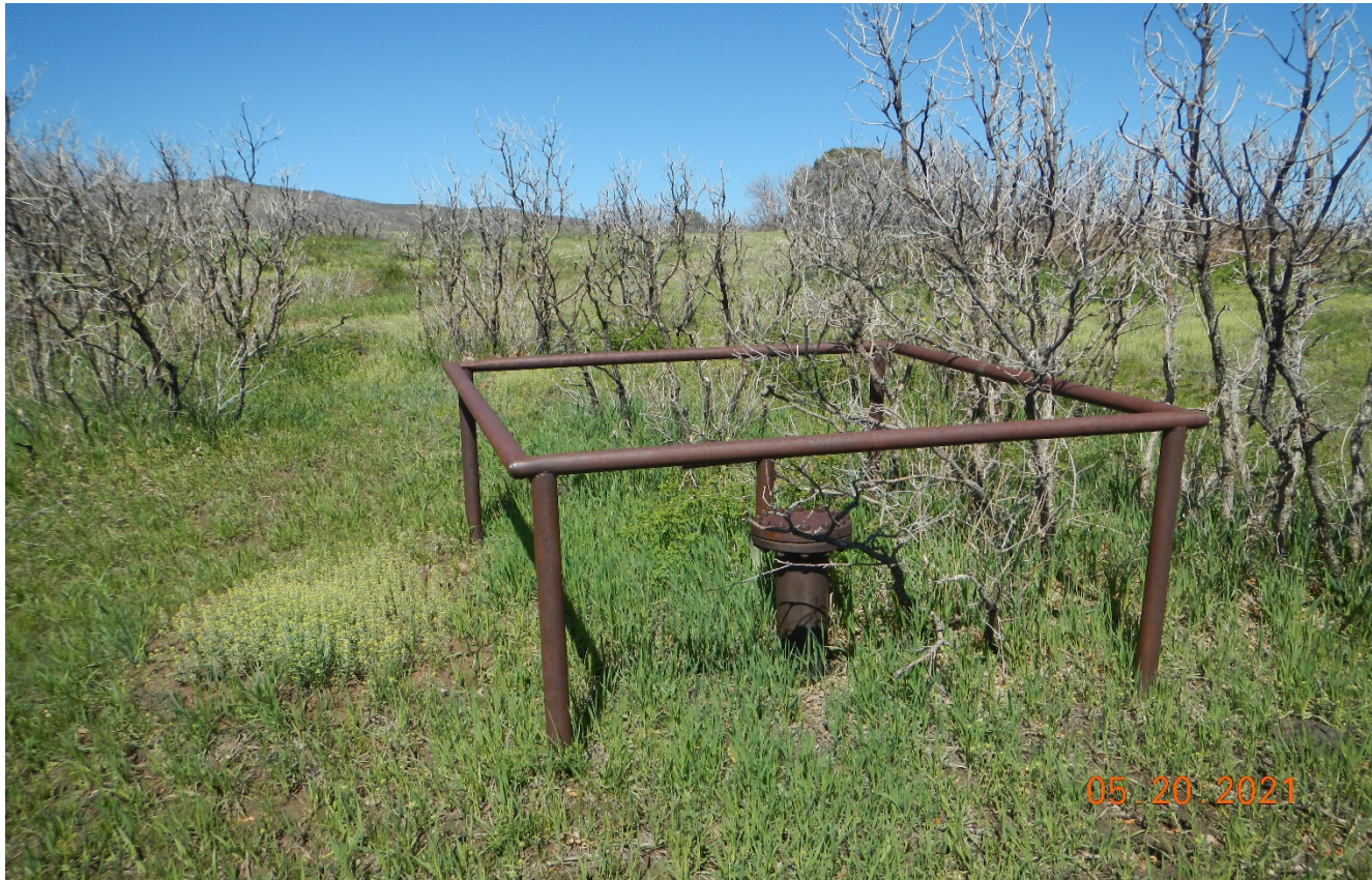
Photo 2. There is a pipeline riser found near the location at Lat/Long:37.4573,-105.05637. All equipment should have been removed within 3 months of plugging the well.
