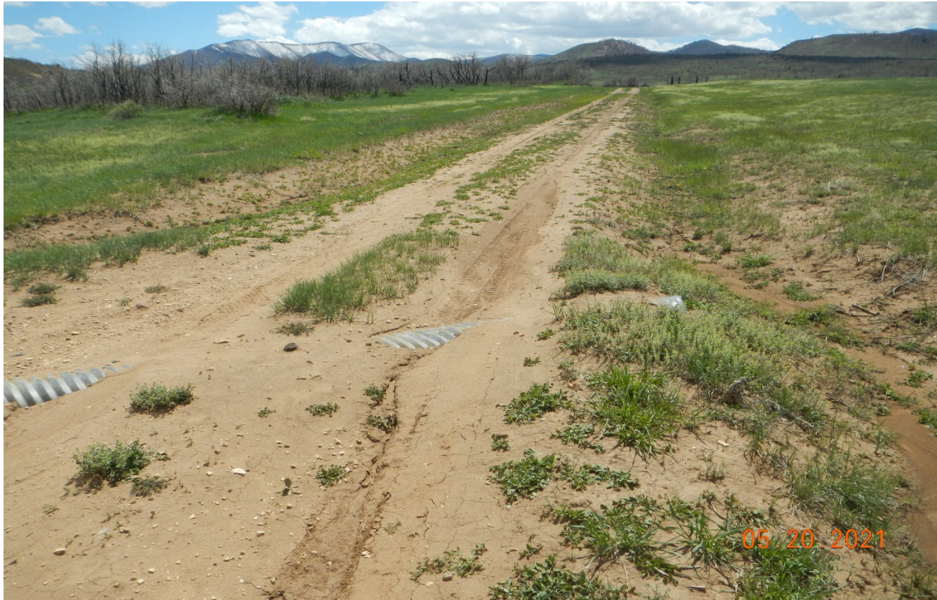
Photo 2. The culvert installed along the access road is not maintained and stormwater is bypassing the culvert. Lat/Long:37.50521,-105.07444.
