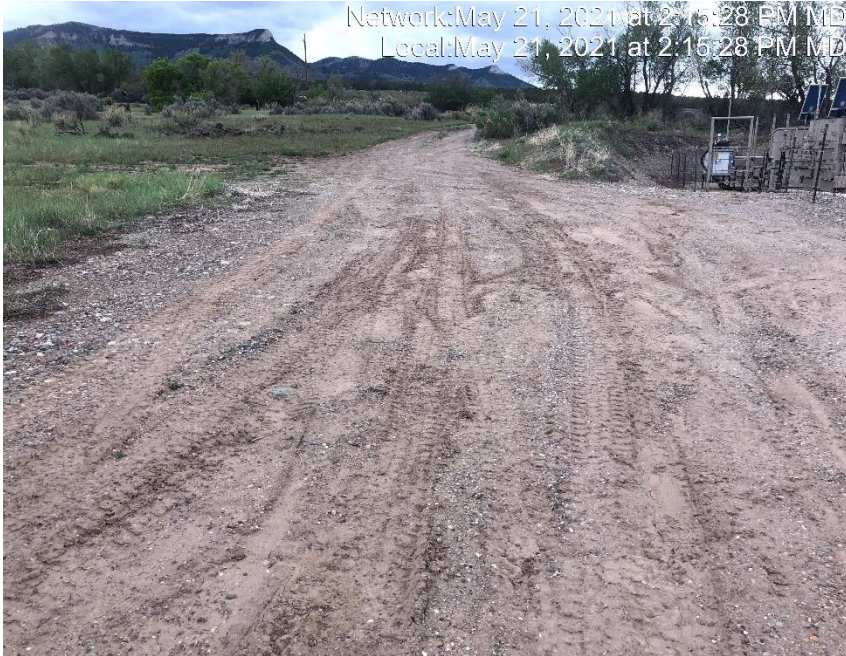
Photo #3903 No form of tracking BMP located at the entrance to location.
