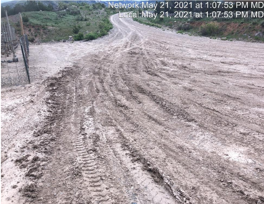
Photo #3892 Location lacks stabilization.
