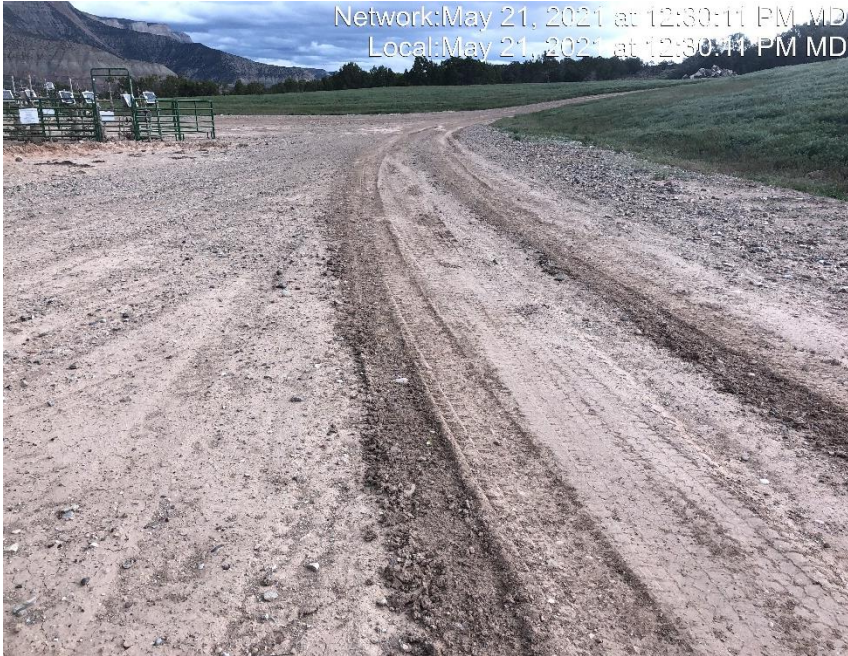
Photo #3888 No form of tacking BMP located at the entrance to location.
