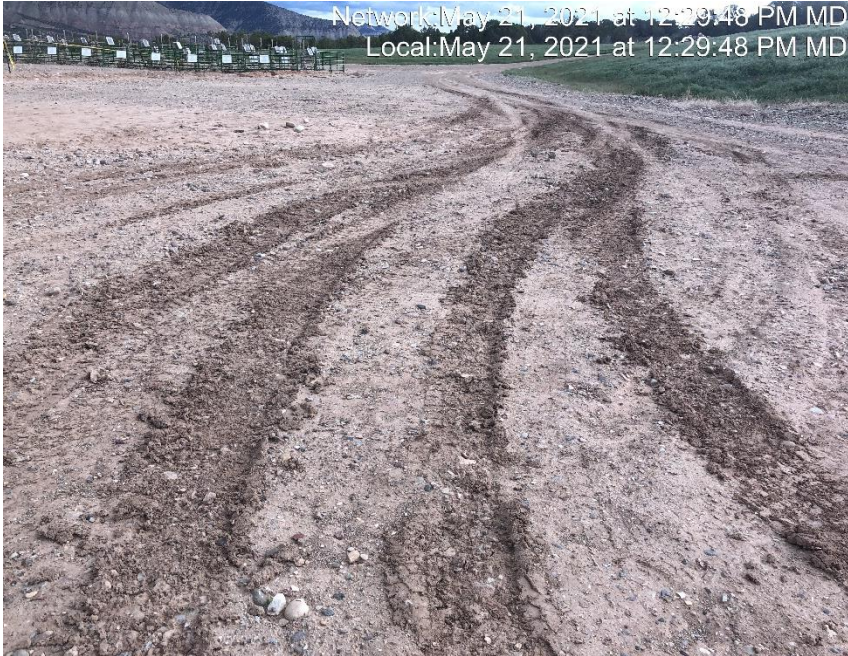
Photo #3887 Location lacks stabilization.
