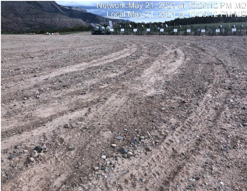
Photo #3886 Location lacks stabilization.
