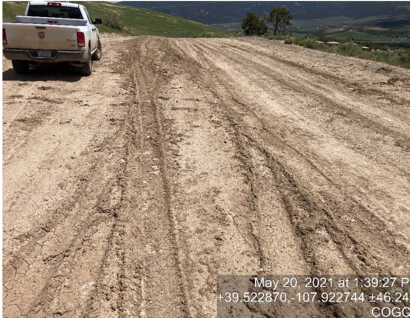
Lack of stabilization/compaction
