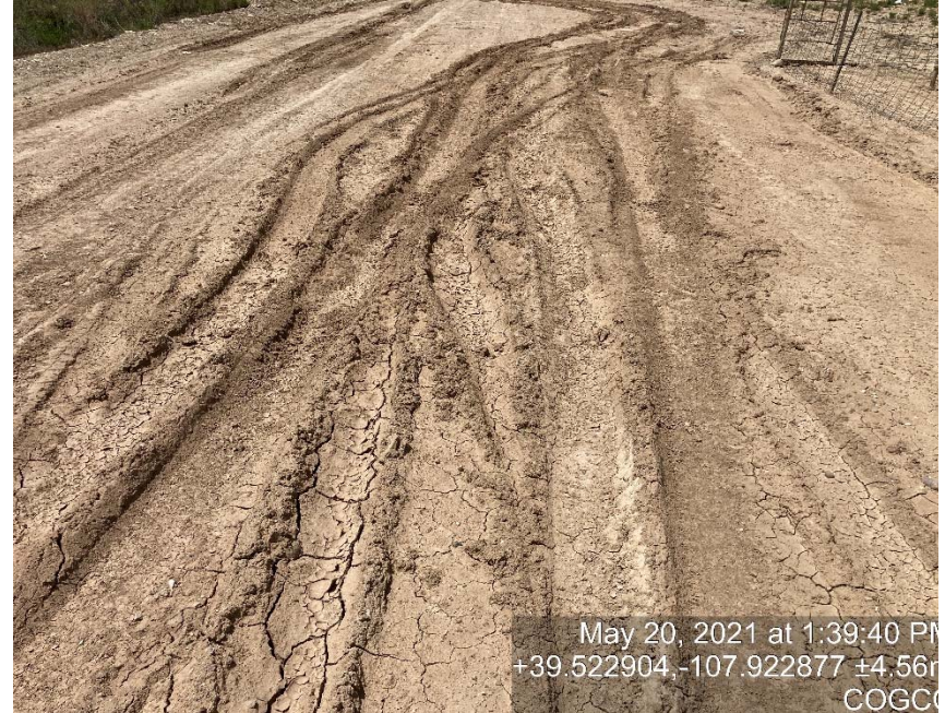
Lack of stabilization/compaction
