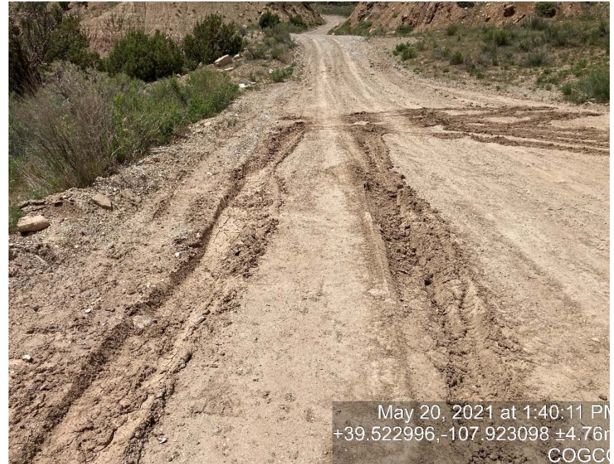
Lack of stabilization/compaction
