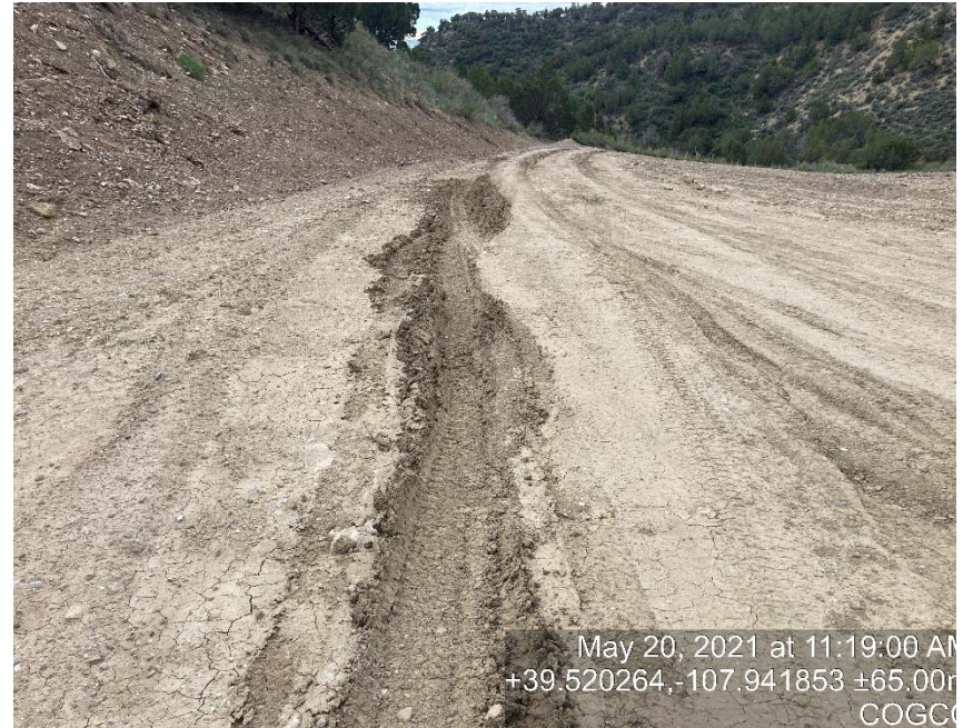
Lack of stabilization/compaction
