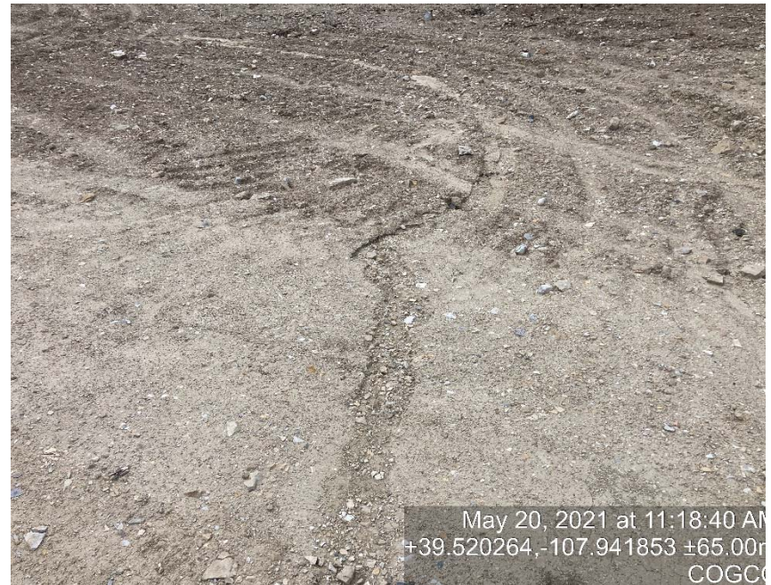
Lack of stabilization/compaction/riling off of pad
