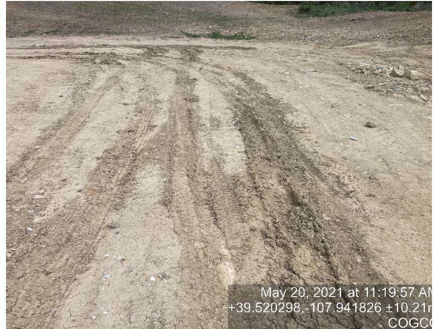
Lack of stabilization/compaction
