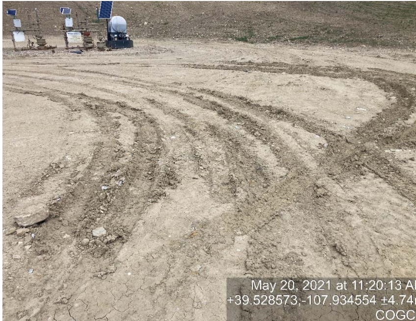
Lack of stabilization/compaction
