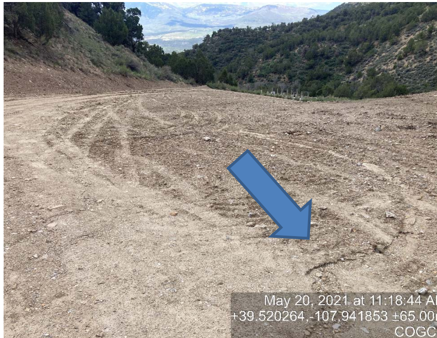
Lack of stabilization/compaction/riling off of pad
