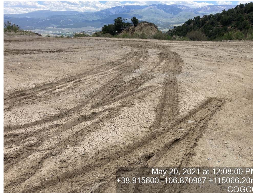
lack of stabilization/compaction
