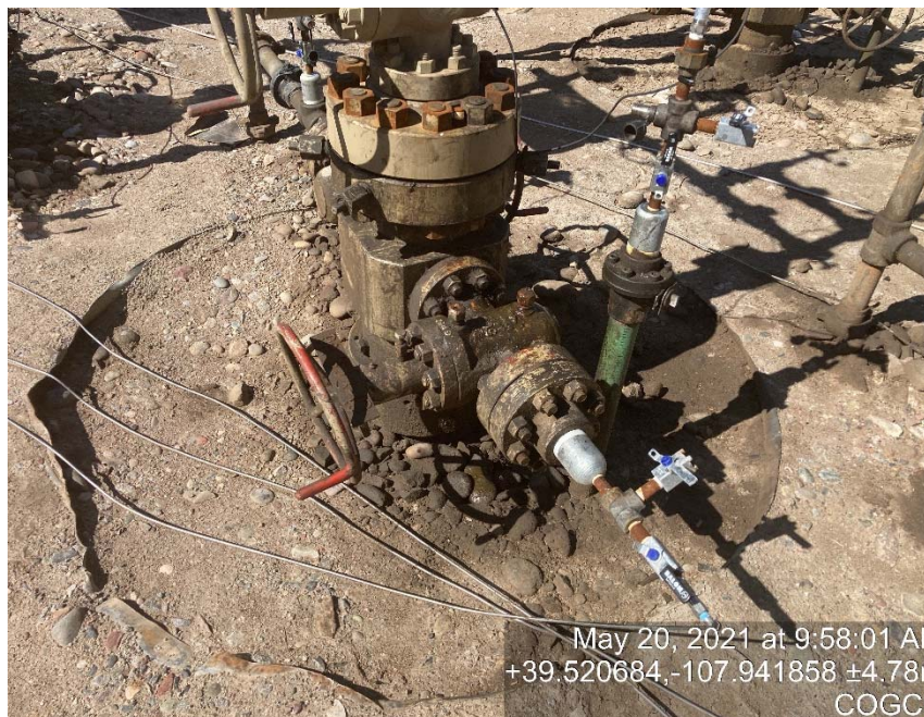
Leaking valve/staining
