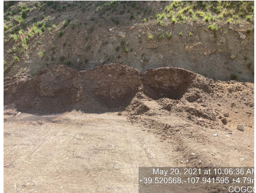
Spoils/cuttings still on location with out containment
