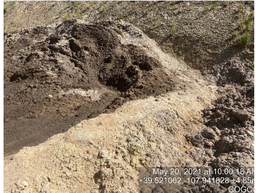
Spoils/cuttings still on location falling out of earth containment
