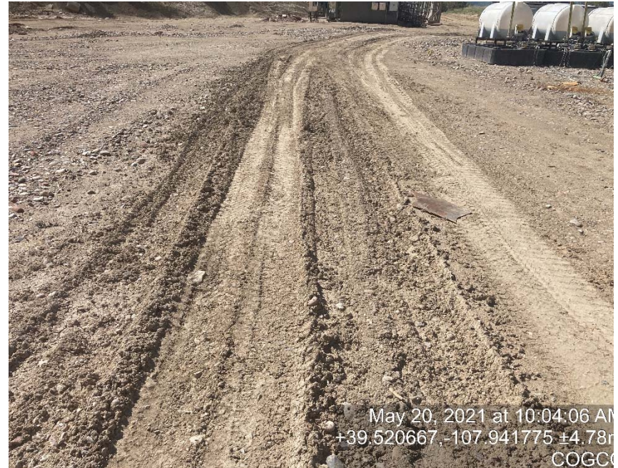
Lack of stabilization/compaction
