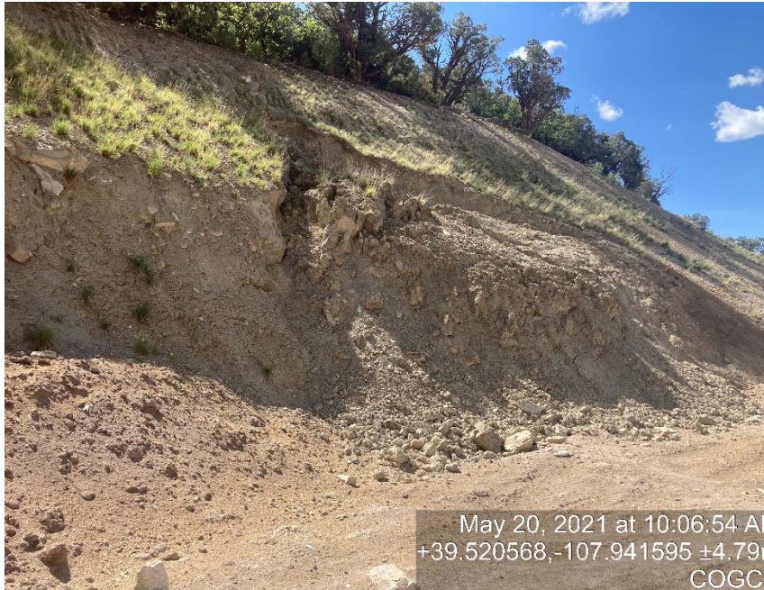
S/E side of location is sluffing no stabilization
