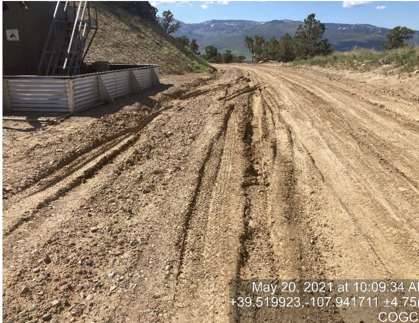
Lack of stabilization/compaction
