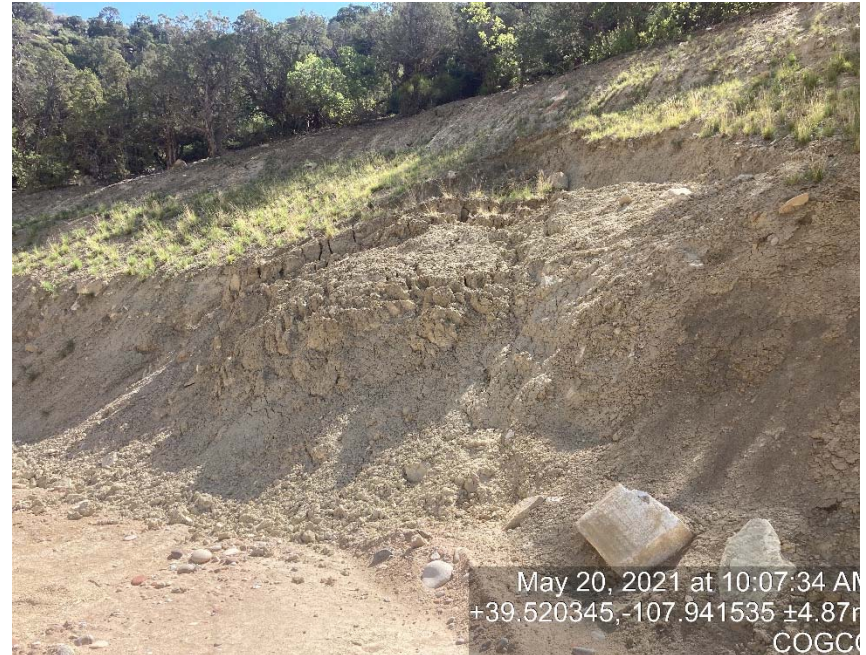
S/E side of location is sluffing no stabilization
