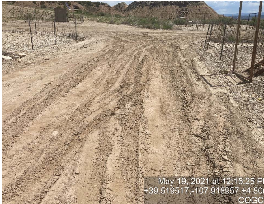
Lack of stabilization/compaction
