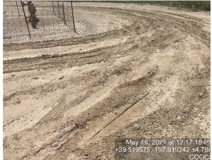
Lack of stabilization/compaction
