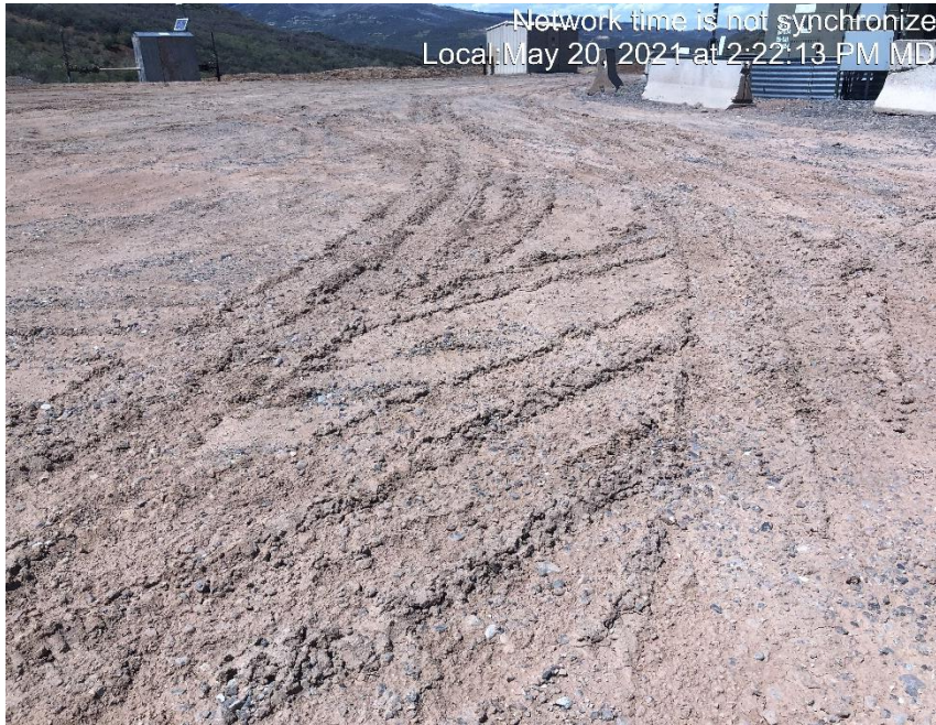
Photo #3879 Location lacks stabilization.
