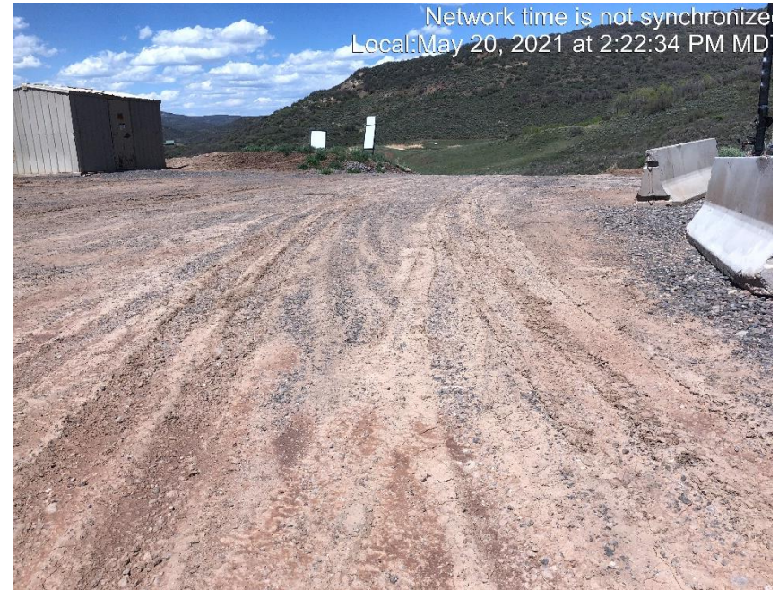
Photo #3880 No form of tracking BMP located at the entrance to location.
