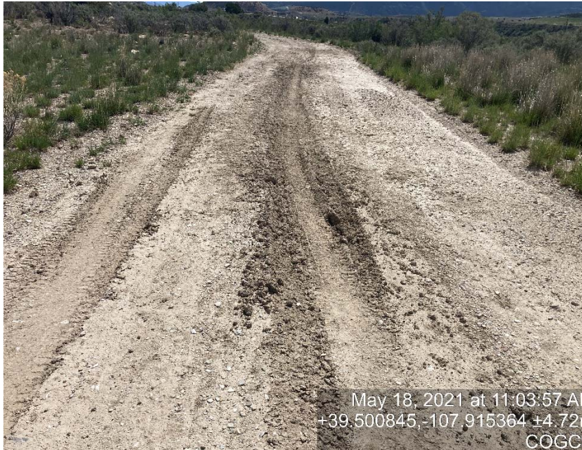
Lack of stabilization/compaction
