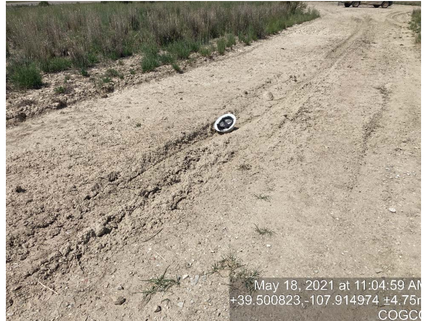
Lack of stabilization/compaction
