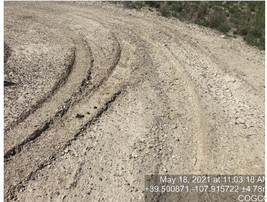
Lack of stabilization/compaction
