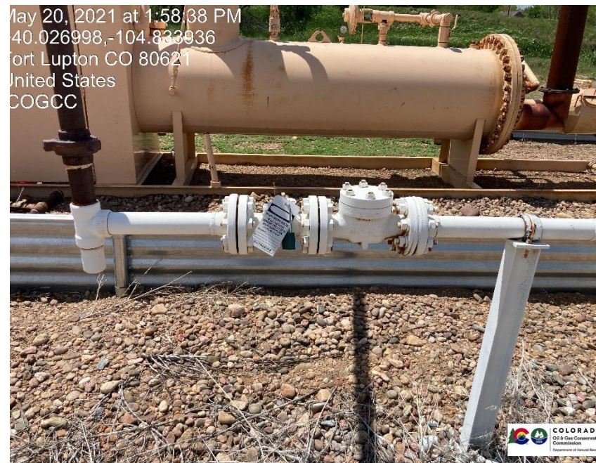
Pic 4 gas line from gas meter run LOTO
