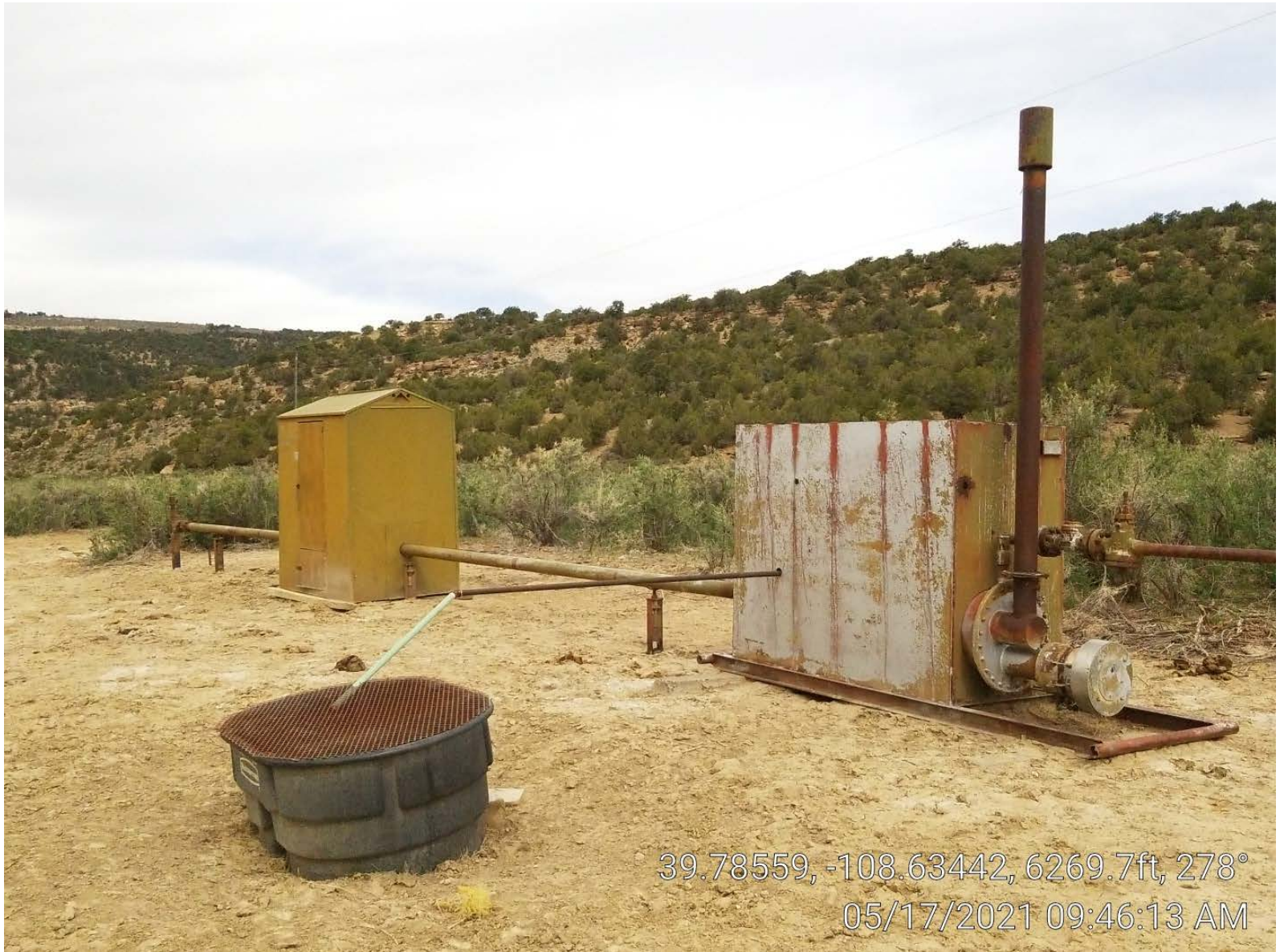
Photo 2. Meter building, tank, separator.
