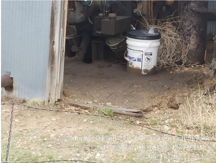
Photo 13 – Stained Soil at Gas Engine
