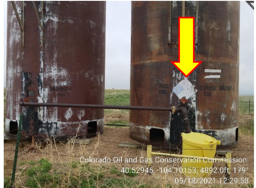
Photo 2 – Tank Battery, NFPA Label Faded
