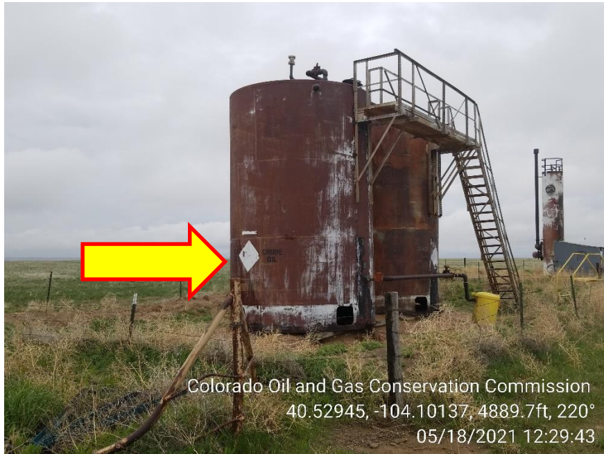
Photo 1 – Tank Battery, NFPA Label Faded
