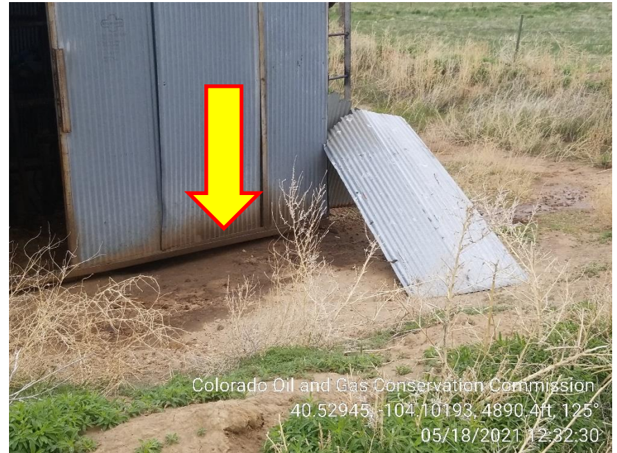
Photo 6 – Stained Soil at Heater Treater
