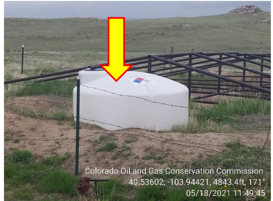
Photo 8 – Capacity Label missing
