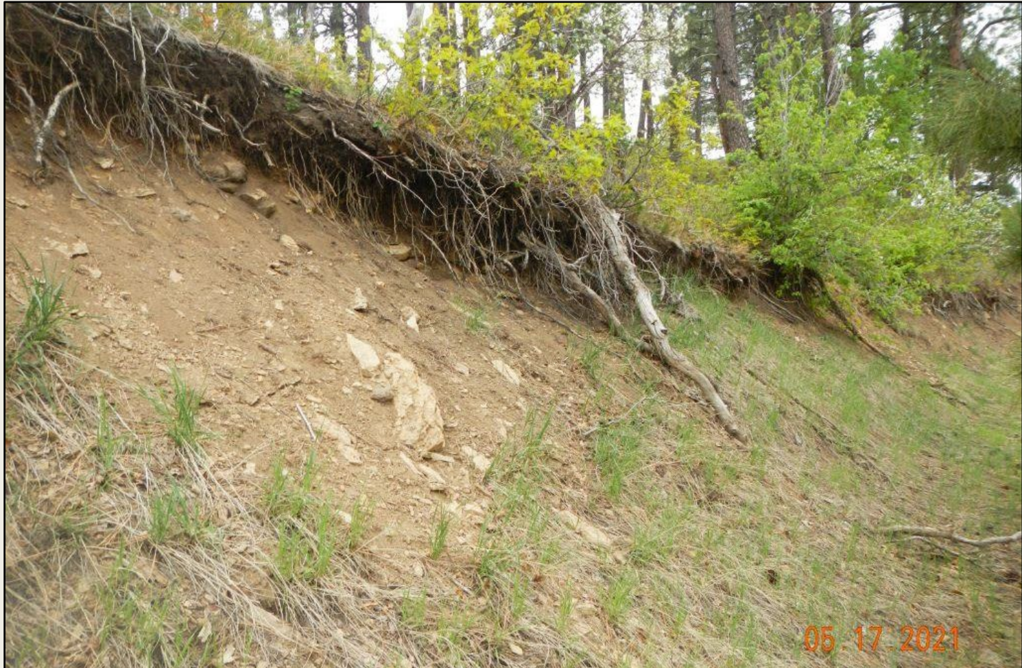
Photo 3. View of erosional downcutting at the top of the eastern cut slope facing. Exposed roots demonstrate lack of stabilization at the top of the cut-slope.
