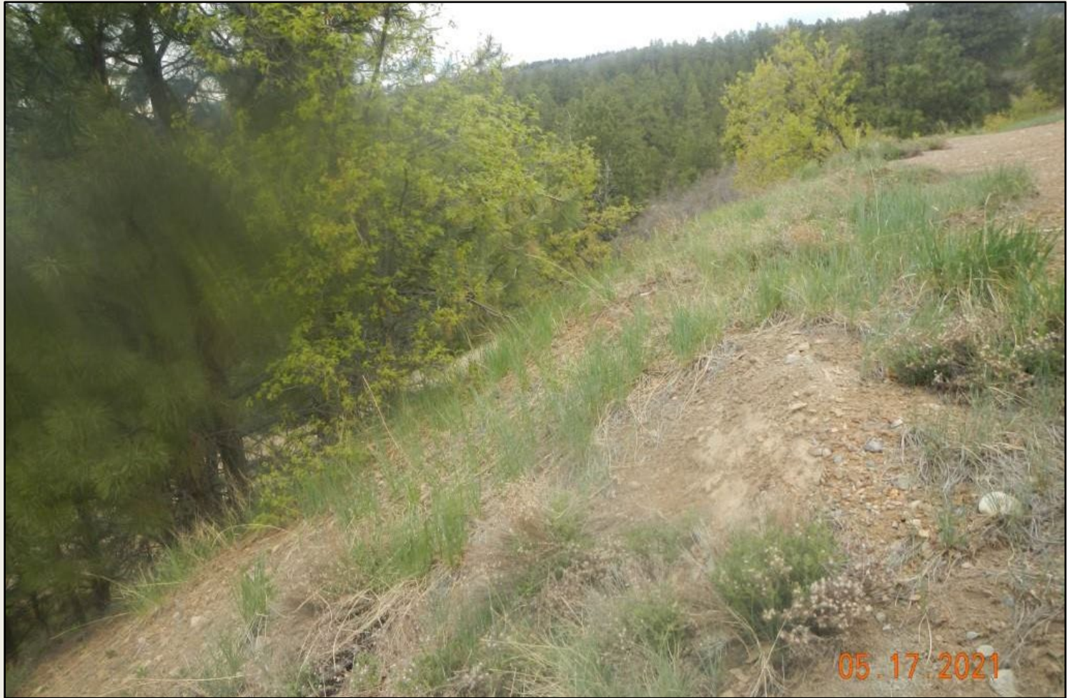
Photo 2. View of the western fill slope from the southwestern corner facing northward. Revegetation is progressing with western wheatgrass, smooth brome, and goldenaster.
