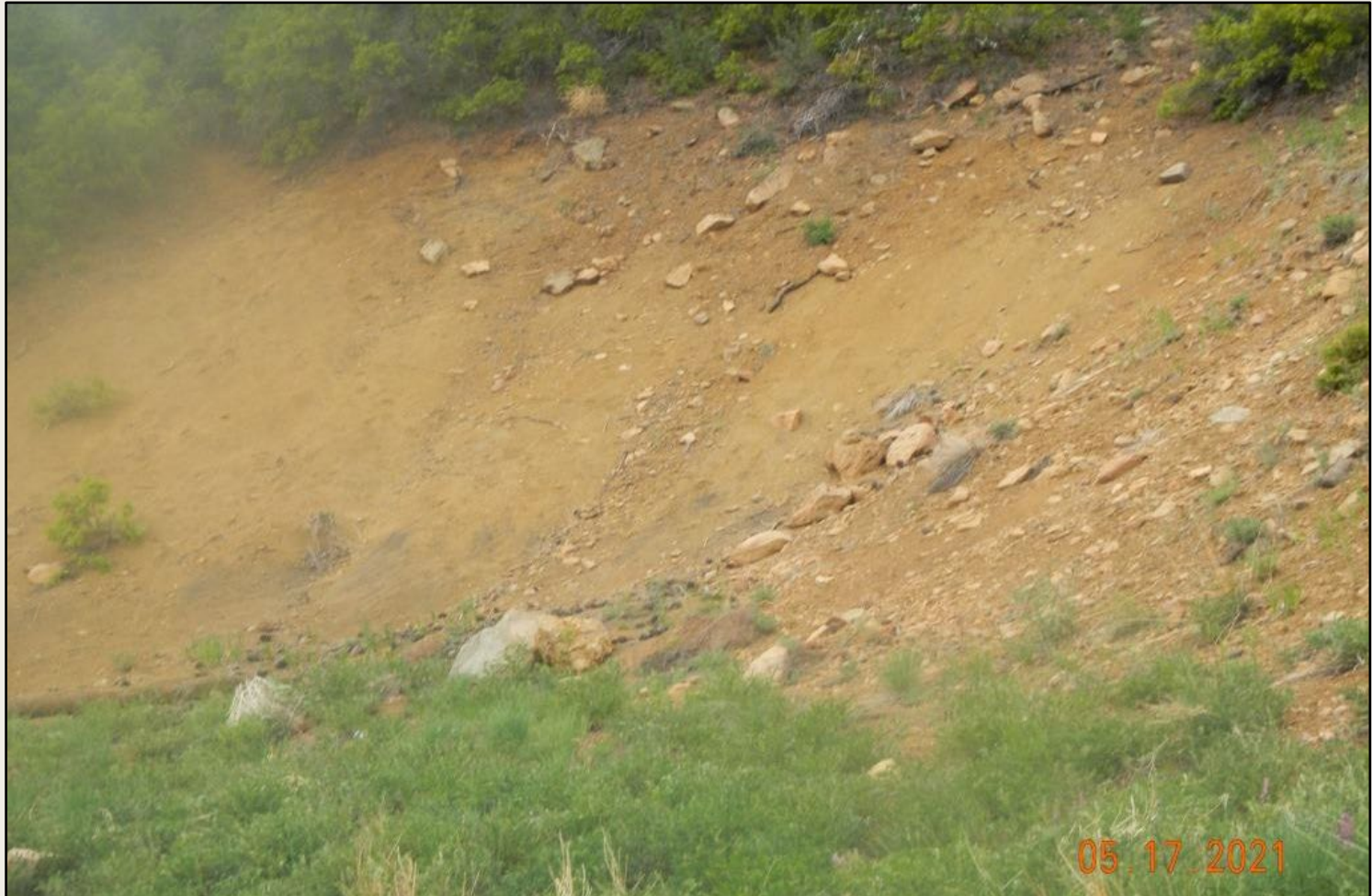
Photo 6. View of cut-slope within the southwestern project area, approximately 30 feet high. Bare soils and little vegetation observed on slope needing recontouring, slope reduction, and stabilization.
