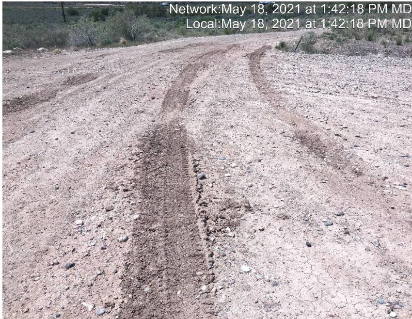
Photo #3855 No form of tracking BMP at entrance to location.
