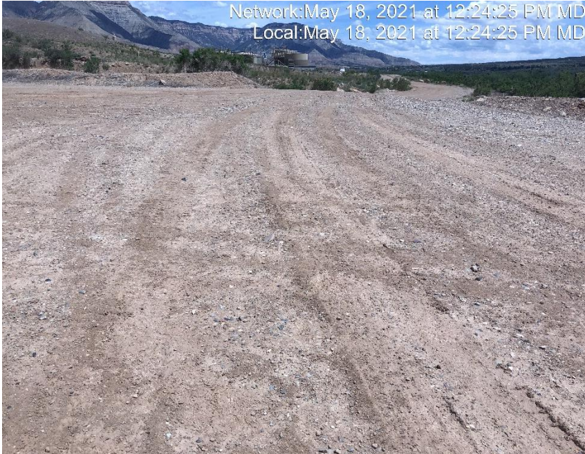
Photo #3842 No form of tracking BMP located at the entrance to location.
