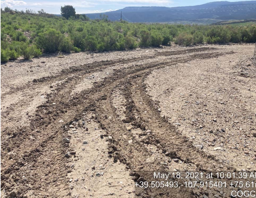
Lack of stabilization/compaction
