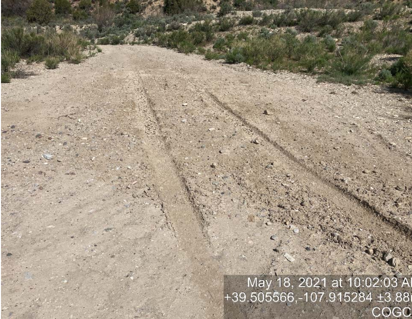
Lack of stabilization/compaction
