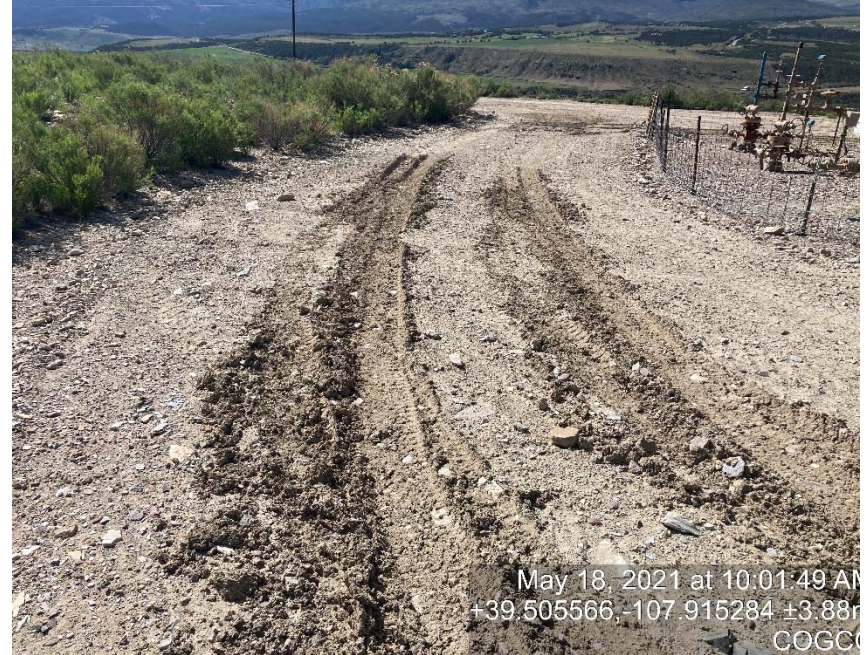
Lack of stabilization/compaction
