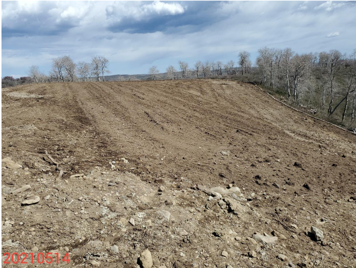
Photo 5: Photo taken from the interim areas on the northeast end of the Location, facing north. Previous inspection required Operator to implement control measures to stabilize the seeded soils. Photo shows that control measures to stabilize the slopes and soils of the interim areas of the Location have not been implemented or maintained.
