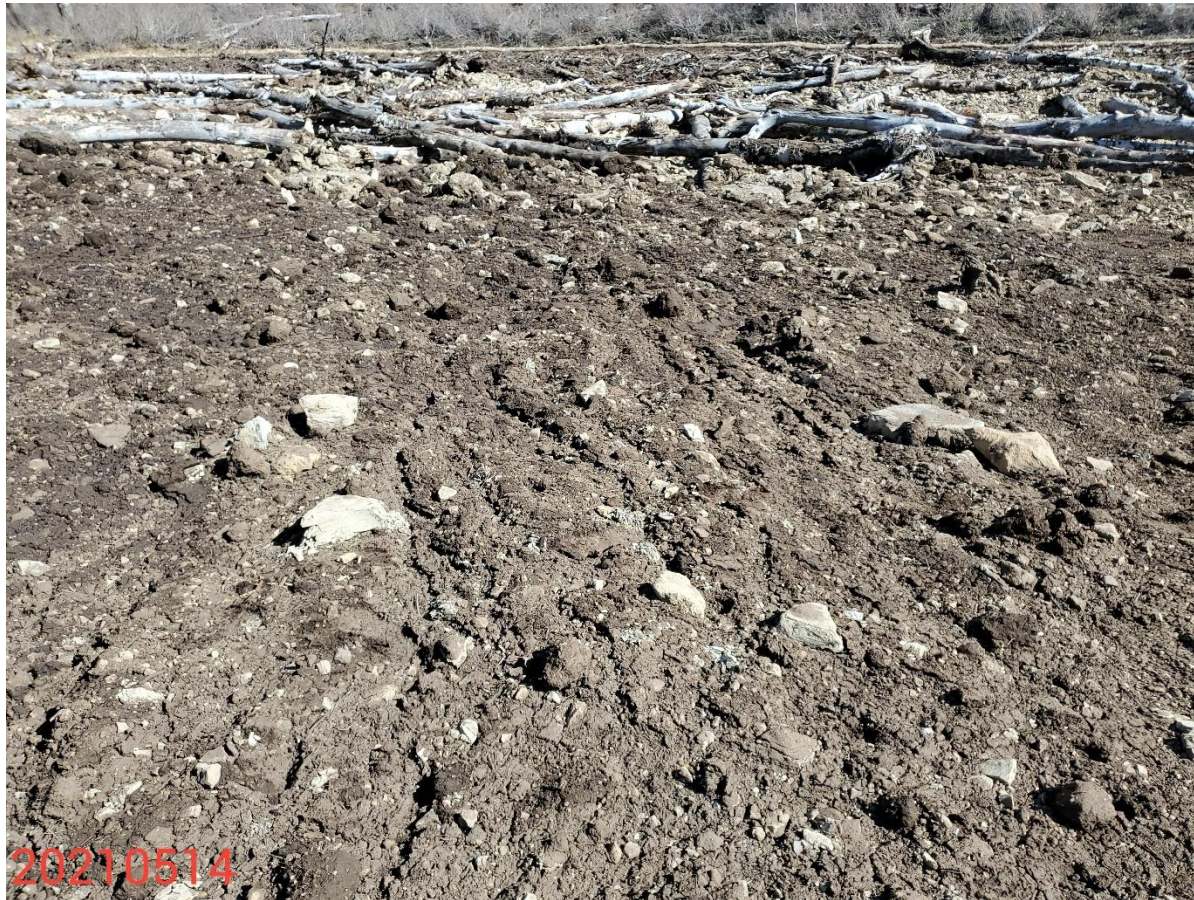
Photo 9: See comments under photo 8. Photo shows stormwater erosion degradation (rilling) observed on interim areas.
