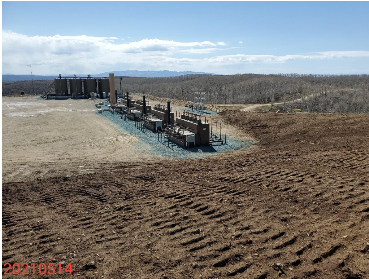
Photo 11: Photo taken from the former cut slope on the west end of the Location, facing southeast. Surface roughening (tracking) observed on western slopes of the Location.
