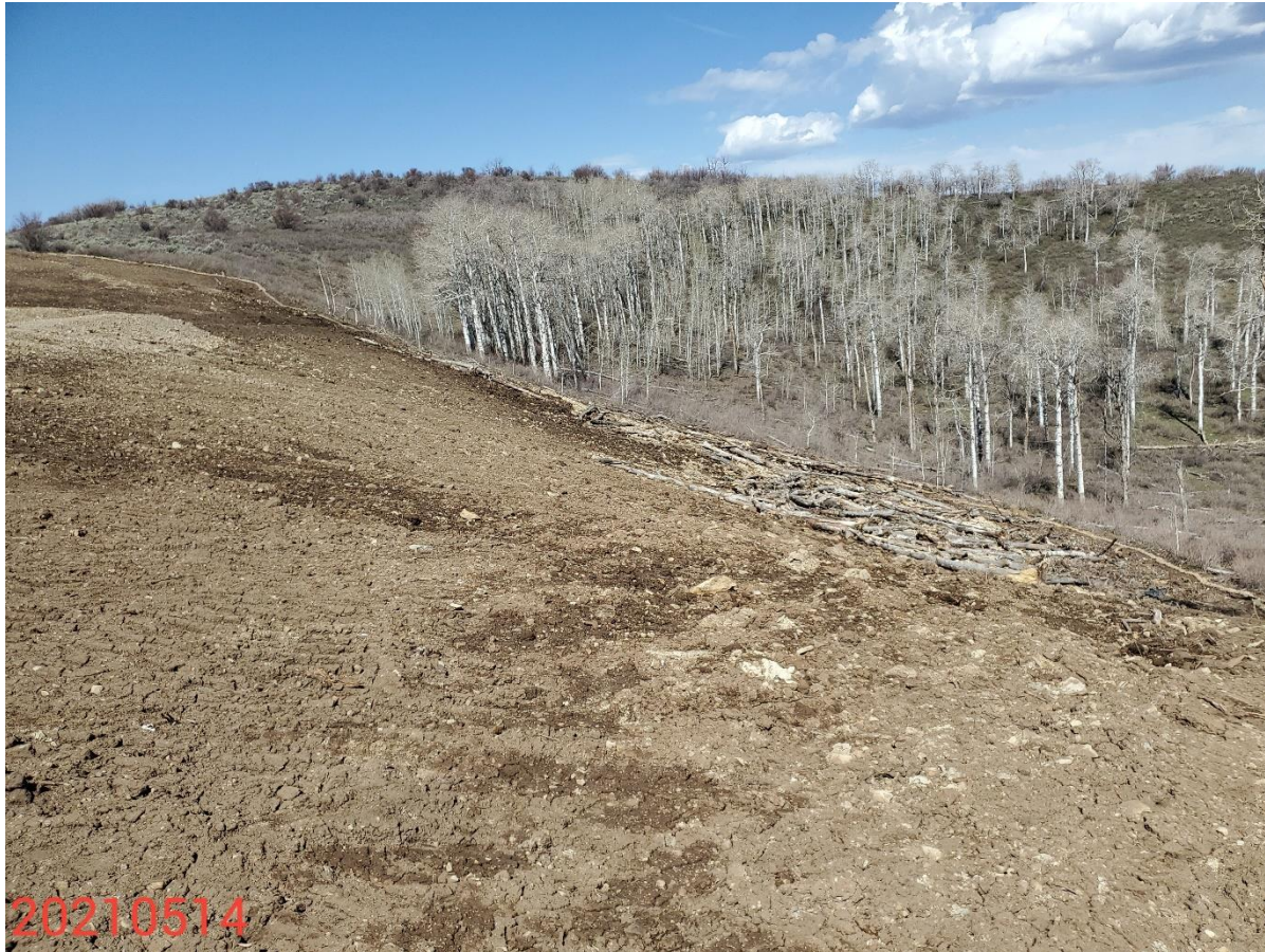
Photo 7: Photo taken from the interim areas on the north end of the Location, facing west. Previous inspection required Operator to implement control measures to stabilize the seeded soils. Photo shows that control measures to stabilize the slopes and soils of the interim areas of the Location have not been implemented or maintained.
