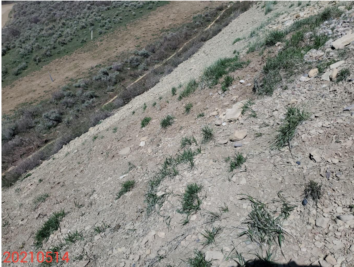
Photo 12: Photo taken from the fill slopes on the southeast end of the Location. Photo shows BMPs to protect/stabilize the fill slopes of the Location remain missing or insufficient.
