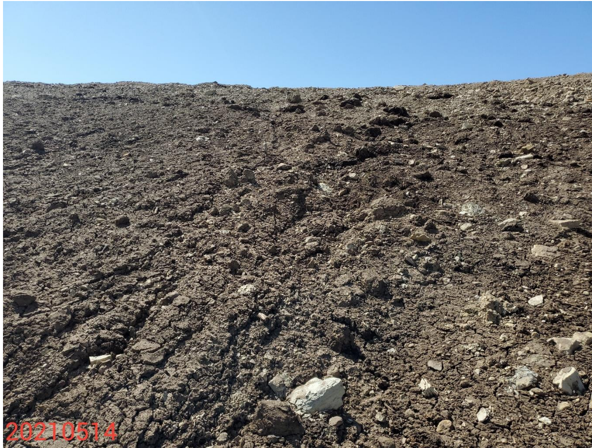
Photo 8: Continued from photo 7. Photo shows erosion degradation (rilling) observed on interim areas. Previous inspection required Operator to implement control measures to stabilize the seeded soils; control measures to stabilize the slopes and soils of the interim areas of the Location have not been implemented or maintained.
