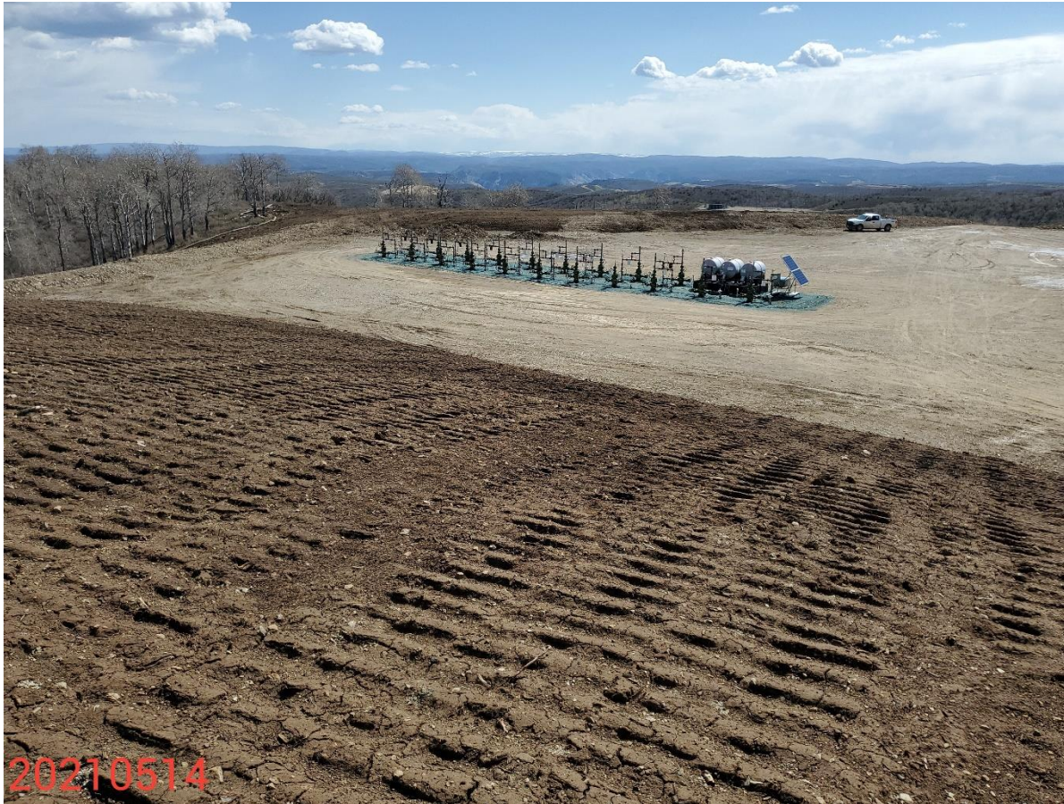
Photo 10: Photo taken from the former cut slope on the west end of the Location, facing northeast. Surface roughening (tracking) observed on western slopes of the Location.
