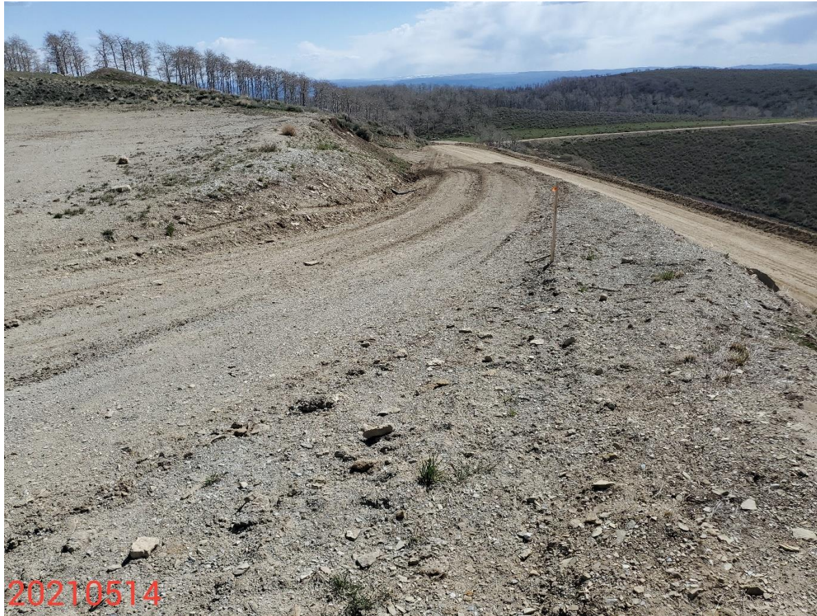
Photo 9: See comments under photo 7. Previous inspection documented that two access points/roads have been constructed on the south end of the Location; inspection required Operator to reclaim areas on the south end of the Location, including the southern access road/point. Photo also shows access road on the south end of the Location has not been reclaimed.
