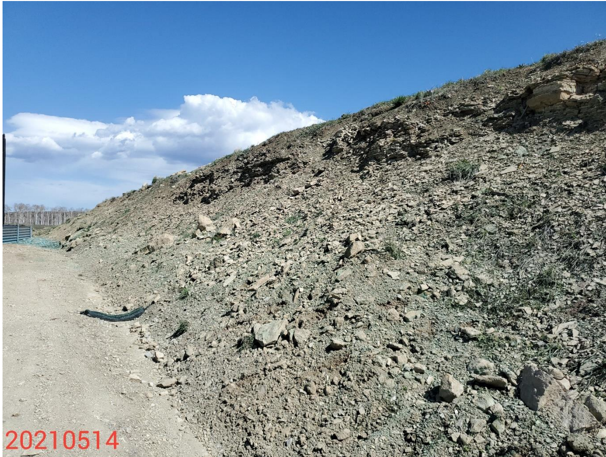
Photo 12: Photo taken from the cut slopes, facing northwest. Previous inspection required Operator to install temporary control measures on slopes until interim reclamation is conducted. Photo shows hydromulch has been applied to slopes; BMP is inadequate for long term stabilization and is showing signs of degradation.
