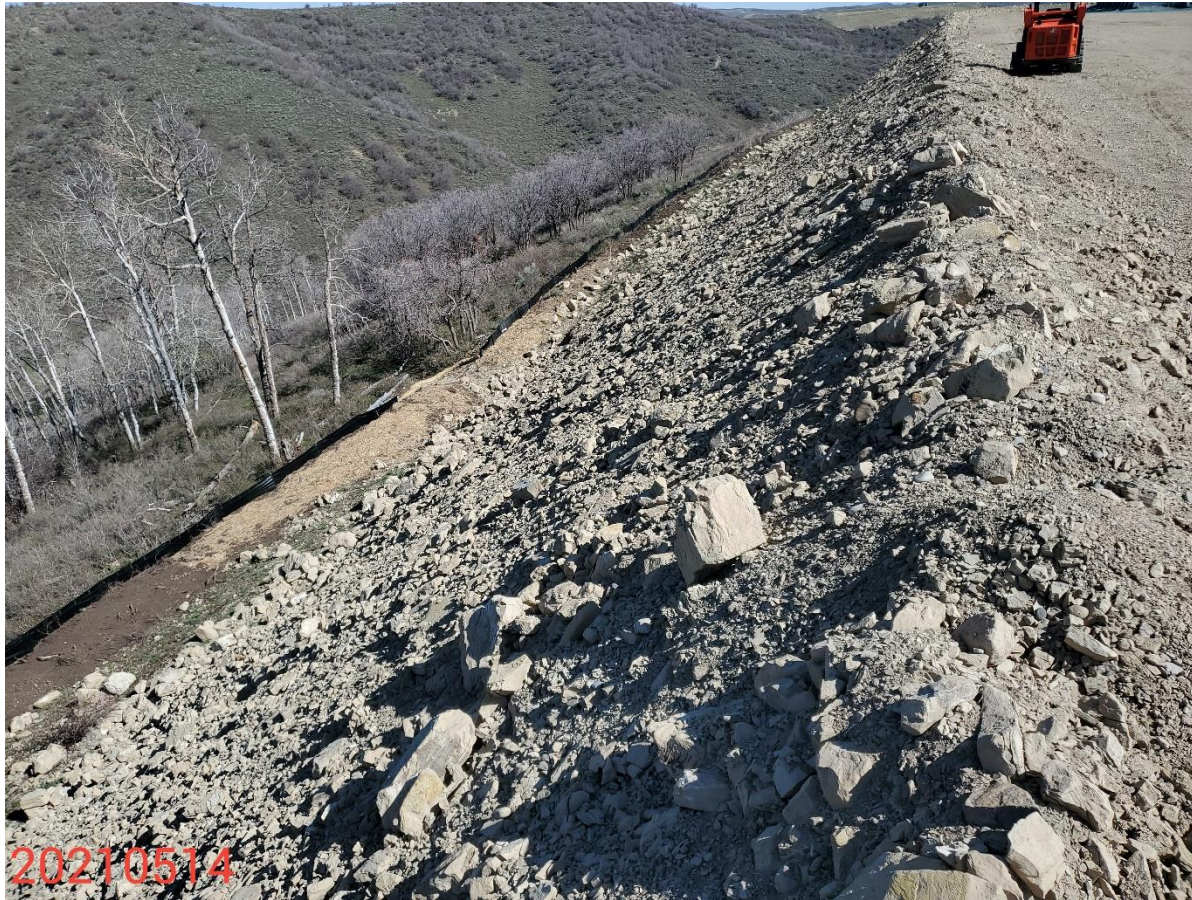
Photo 5 Photo taken from the west end of the Location, facing north. Photo shows Operator has maintained perimeter control measures to manage stormwater runoff from the Location. Photo also shows that required control measures to protect/stabilize the fill slopes on the Location remain missing or insufficient.
