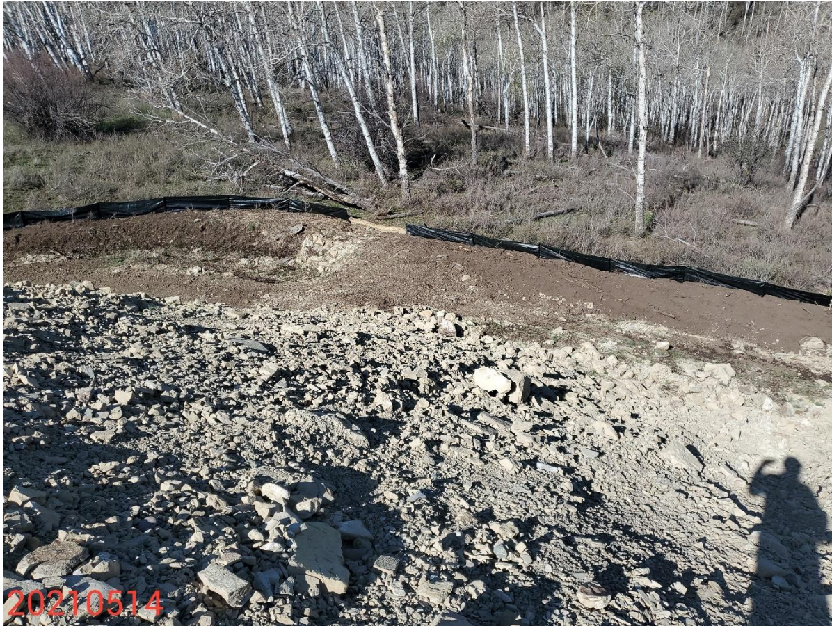
Photo 6: Photo taken from the west end of the Location, facing southwest. Photo shows Operator has maintained perimeter control measures to manage stormwater runoff from the Location. Photo also shows that required control measures to protect/stabilize the fill slopes on the Location remain missing or insufficient.
