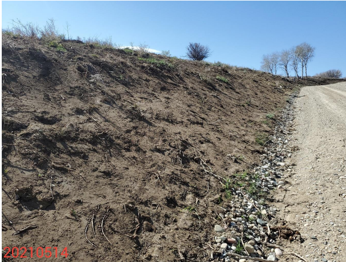
Photo 8: Photo taken from the access road, facing south. Previous inspection required Operator to conduct additional reclamation along the access road, and to implement control measures to stabilize the seeded soils; unable to find evidence that additional reclamation was performed, and control measures installed.
