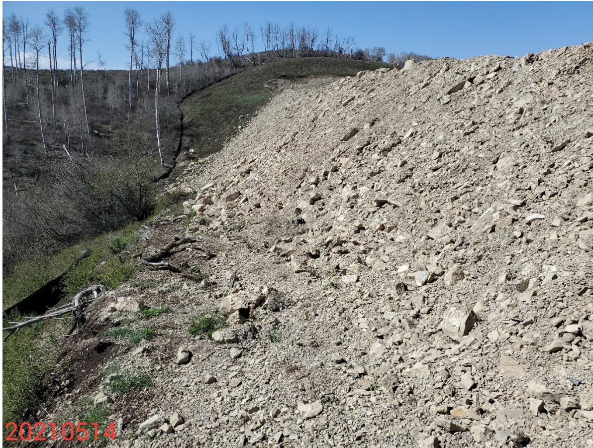
Photo 7: Photo taken from the east end of the Location, facing south. Photo shows that required control measures to protect/stabilize the fill slopes on the Location remain missing or insufficient.
