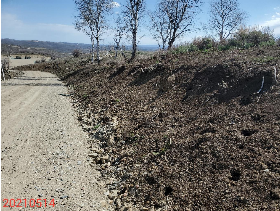
Photo 9: Photo taken from the access road, facing north. Previous inspection required Operator to conduct additional reclamation along the access road, and to implement control measures to stabilize the seeded soils; unable to find evidence that additional reclamation was performed, and control measures installed.
