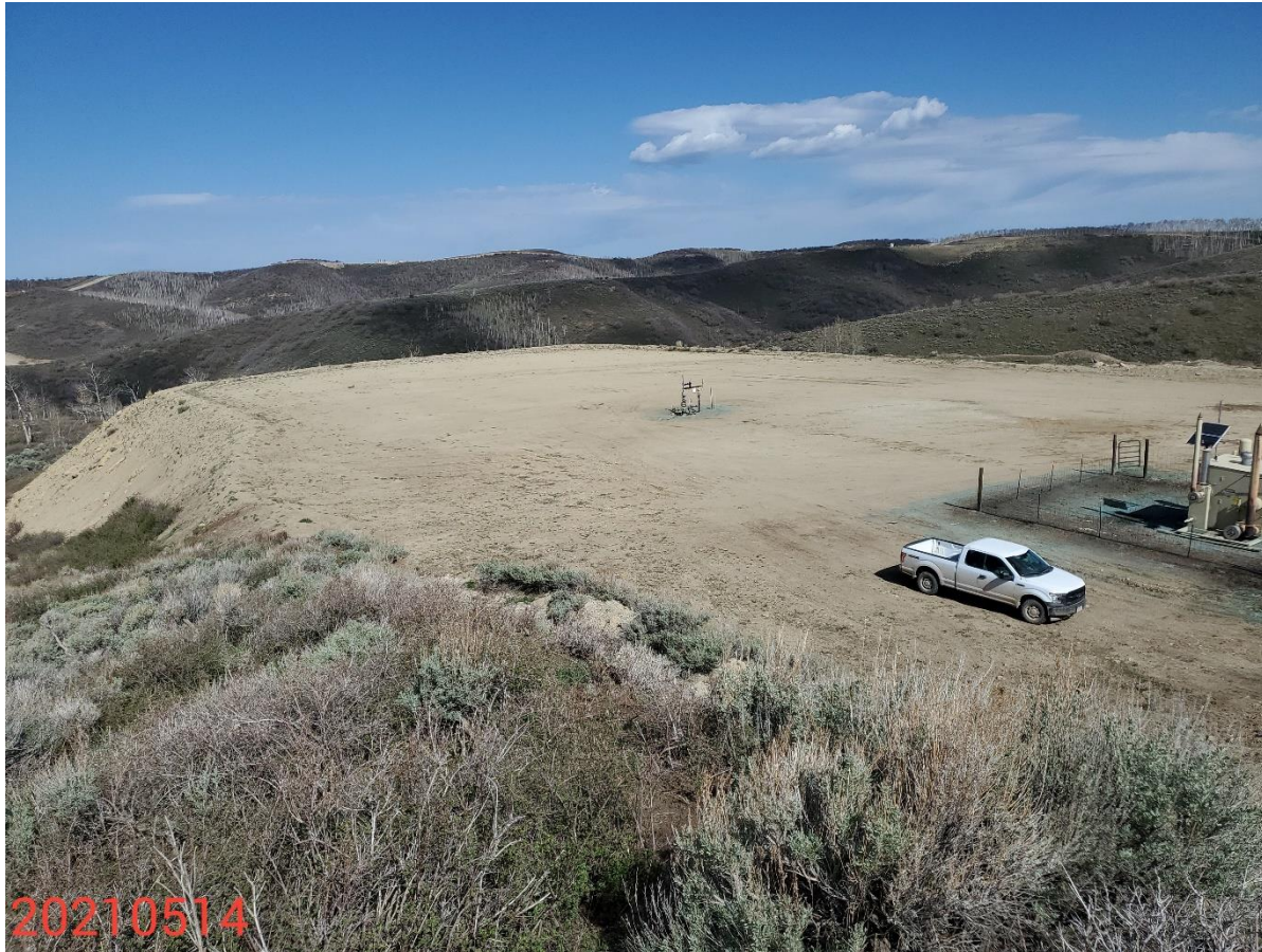
Photo 6: Photo taken from the southeast of the Location, facing northwest. See comments under photo 1. Control measures to protect/stabilize the fill slopes of the Location remain missing or insufficient.
