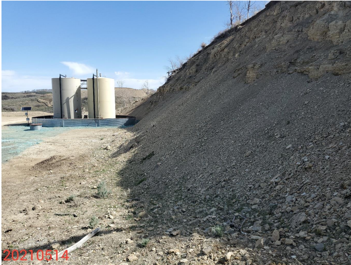
Photo 7: Photo taken from the cut slopes of the Location, facing north. Photo shows control measures to protect/stabilize the cut and fill slopes of the Location remain missing or insufficient.
