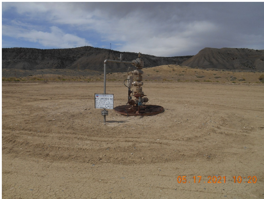
Injection wellhead
