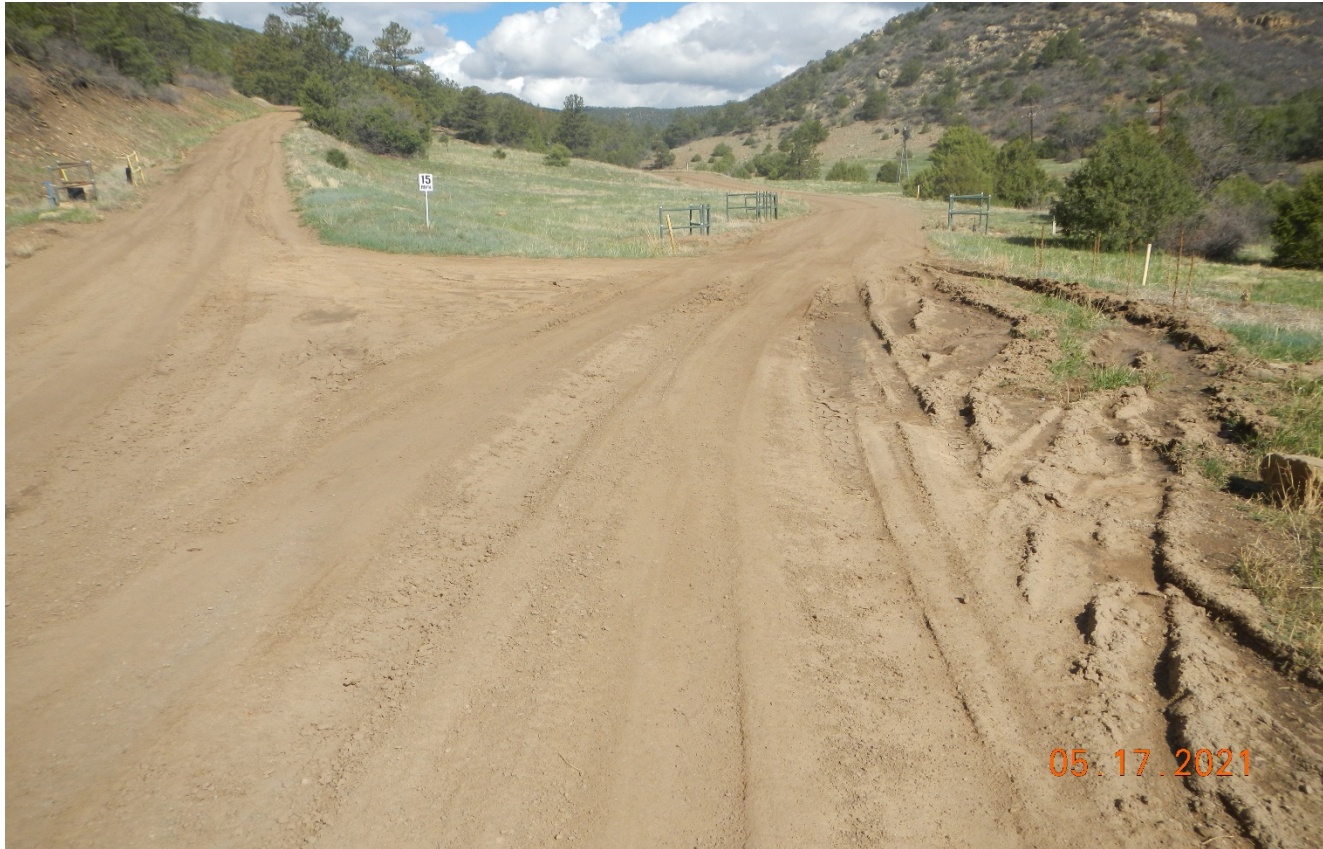
Photo 1. There is vehicle disturbance off the side of the road. The disturbance needs to be reclaimed.
