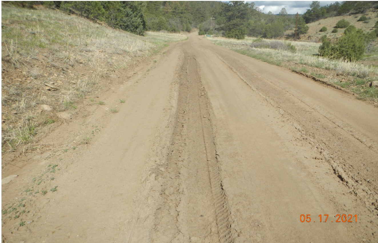
Photo 2. There is vehicle rutting along the main road. Areas of rutting need to be stabilized.
